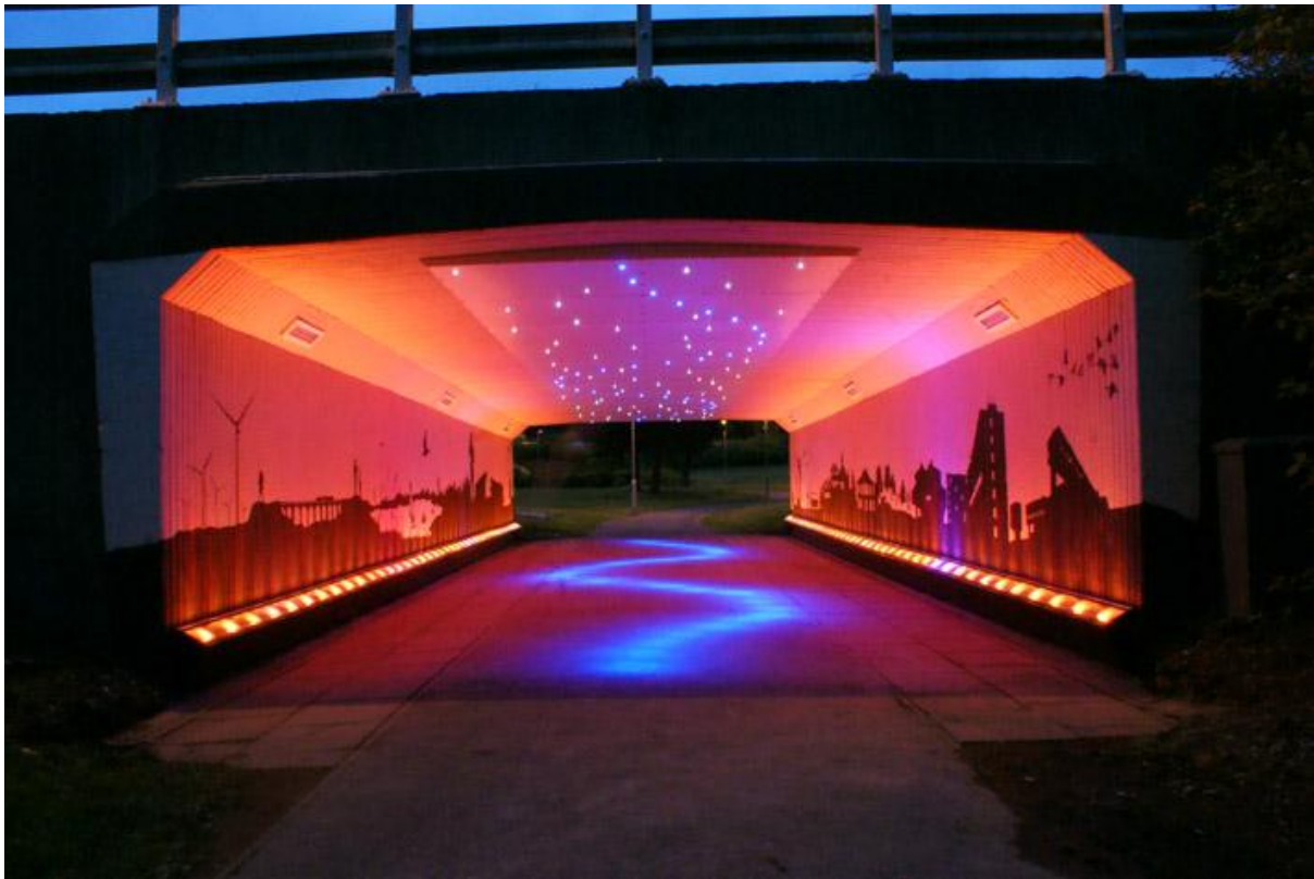
Example of a transformed tunnel, Craiglinn underpass, Cumbernauld, UK
