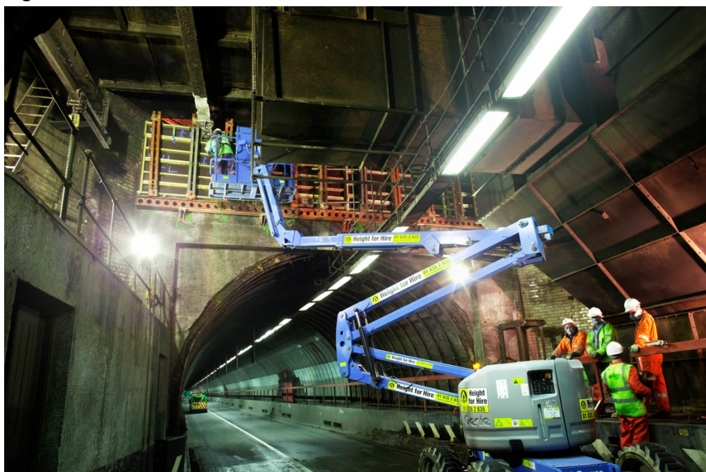
Figure D-12: Maintenance of the northbound tunnel bore
