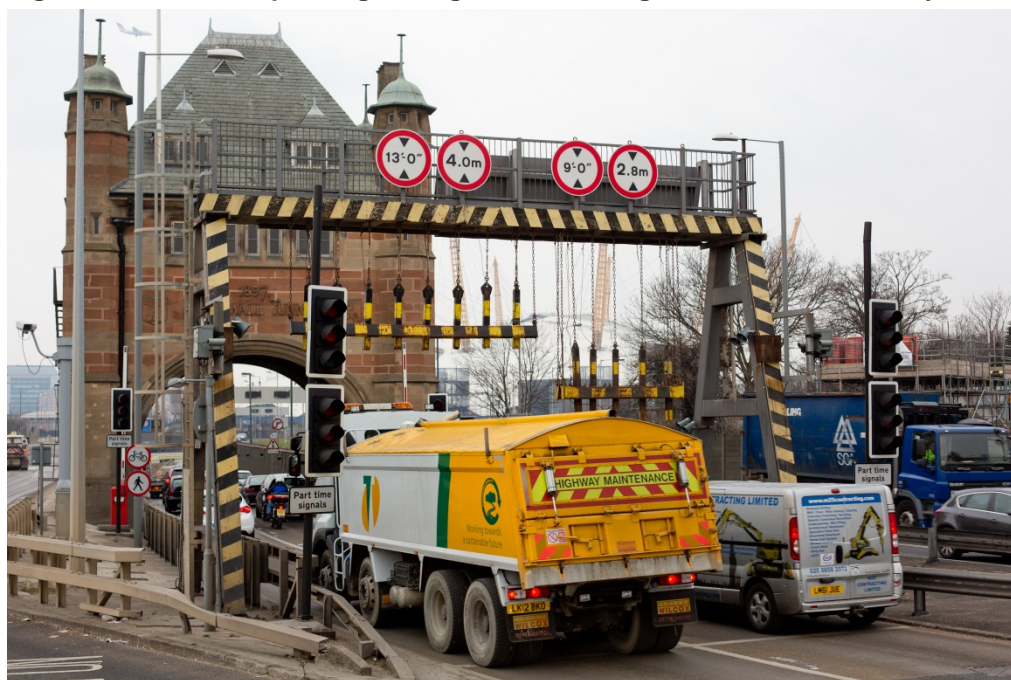
Figure D-6: Vehicles passing through the over height vehicle detection system
