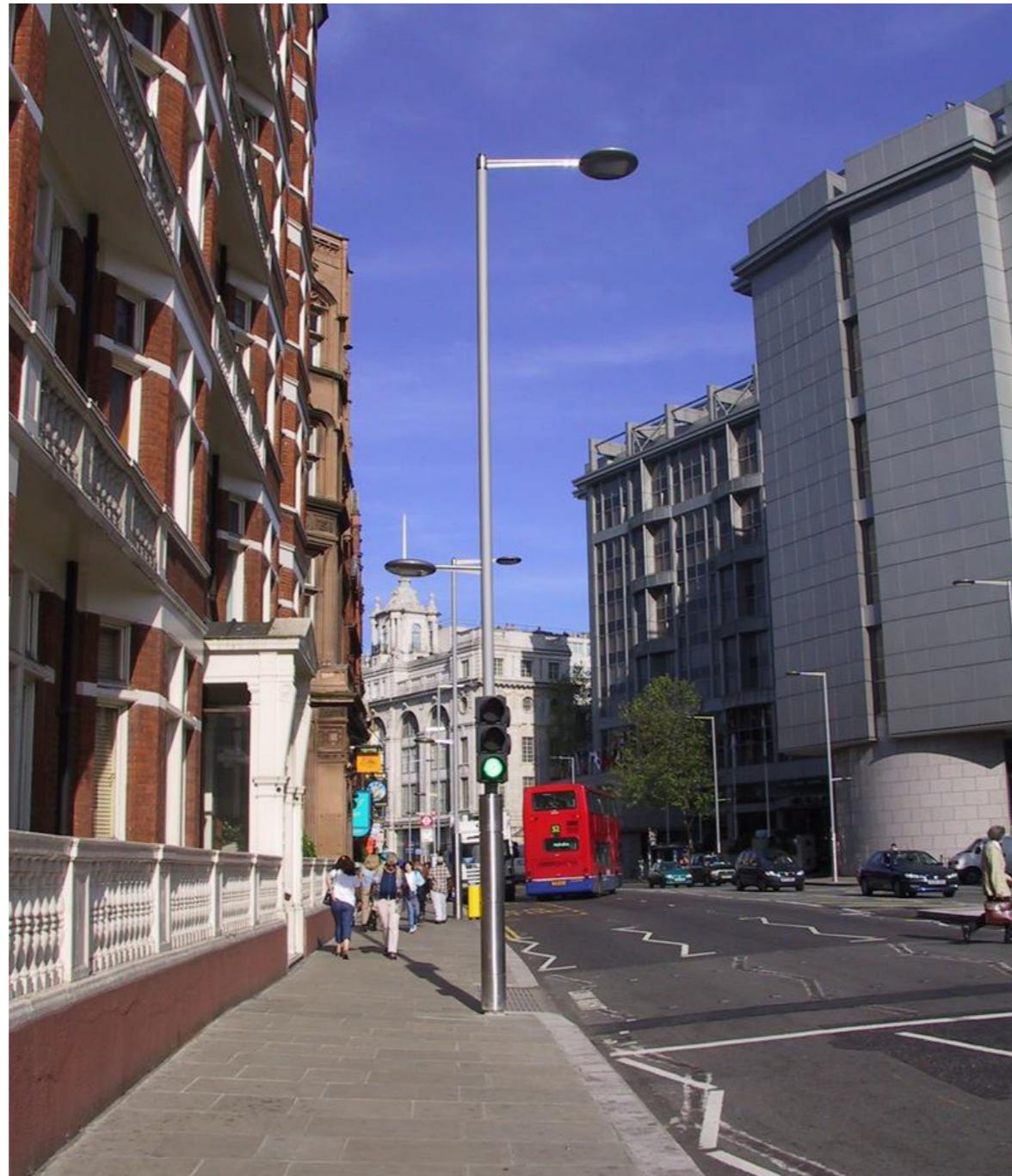
Figure 9.8 Light column with split level highway / footway lighting, and integrated traffic lights.
