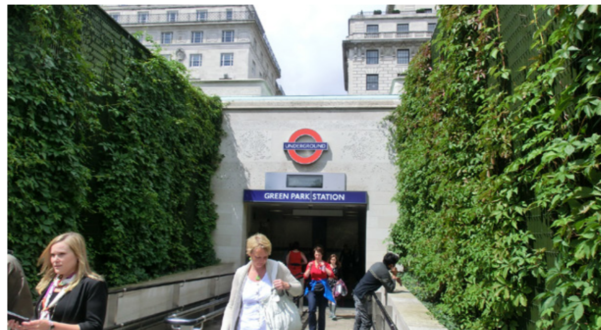
Figure 8.4 Green façade at Green Park Station, London
