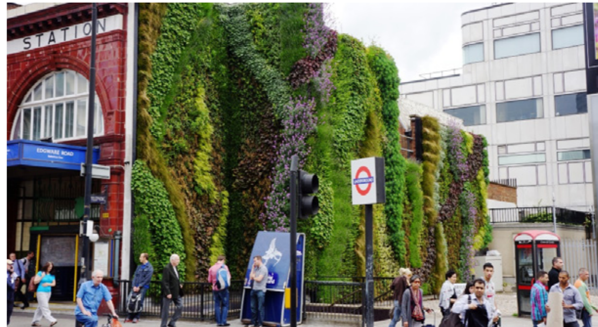
Figure 8.3 Green Wall at Marylebone Road, Edgware Road Station, London
