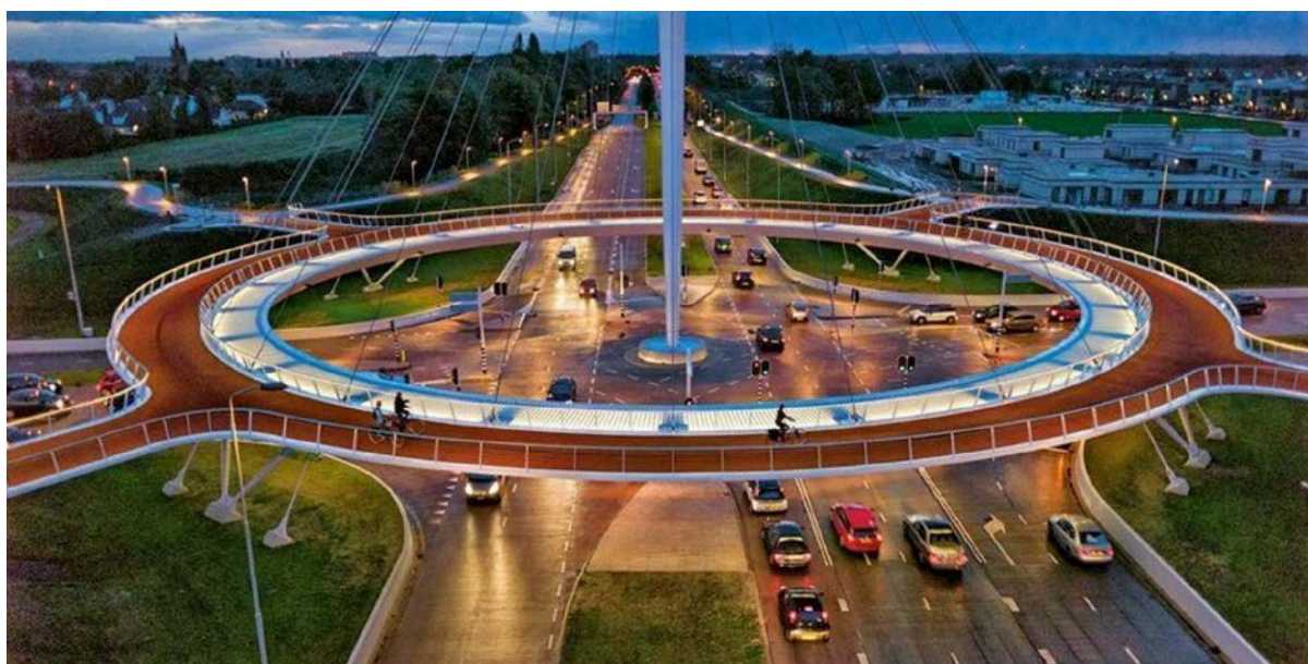
Figure 21: Example of grade separated cycle infrastructure in the Netherlands – the Hovenring
