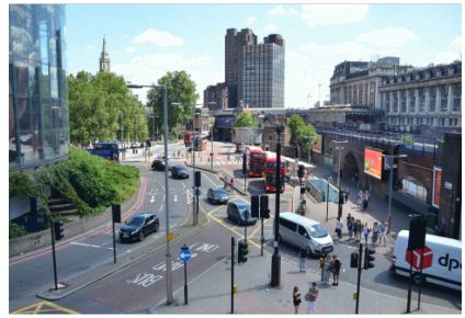
Work will start to transform Waterloo roundabout, making it safer for cyclists, improving crossings and bus interchanges
