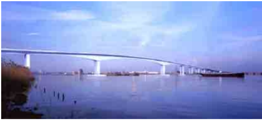
Figure 2.3 – Illustrative Visual of Spine Beam Box Girder
