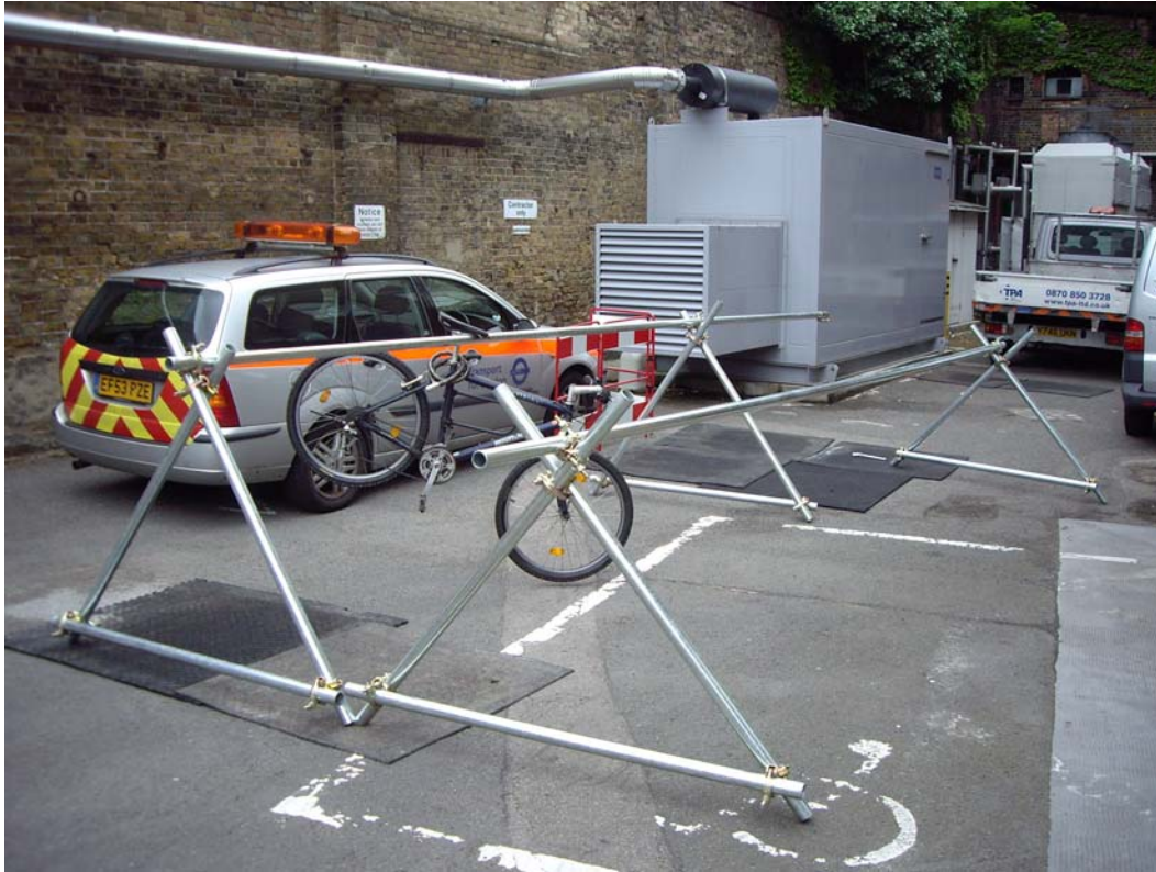
Photo 5: Temporary cycle parking using scaffolding
