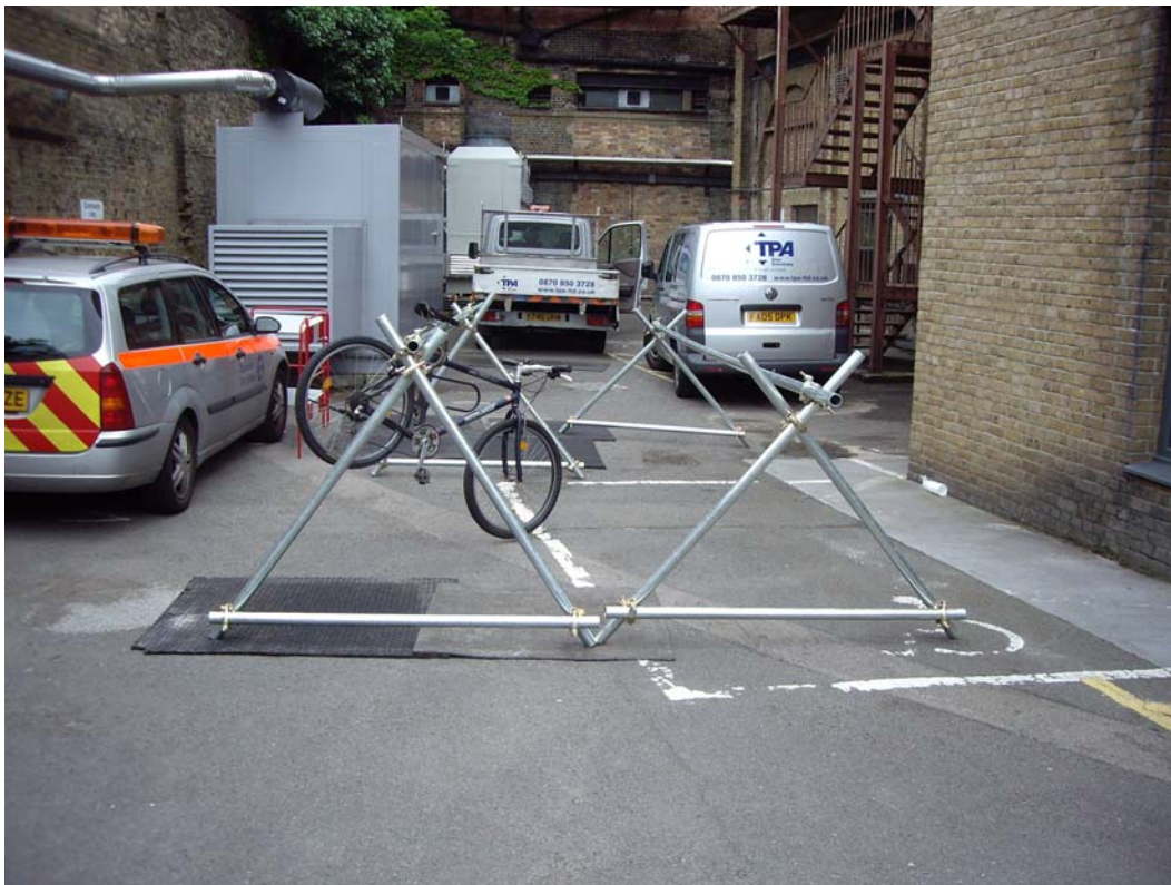
Photo 6: Temporary cycle parking using scaffolding
