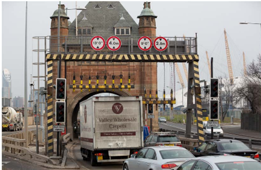
Figure 2-15 Blackwall Tunnel northbound bore height restrictions
