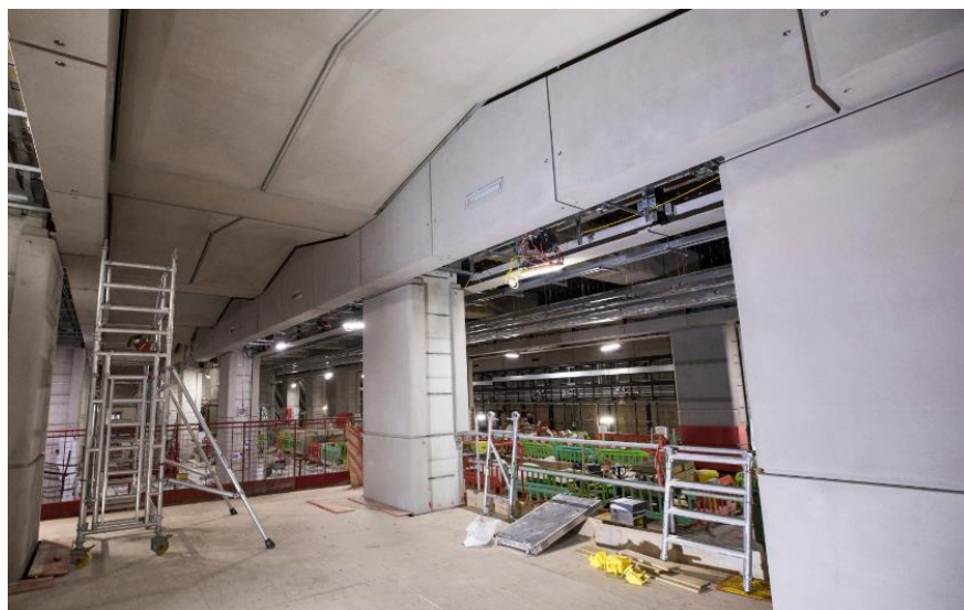
Fig 3. Cladding and tiling at ticket hall level
