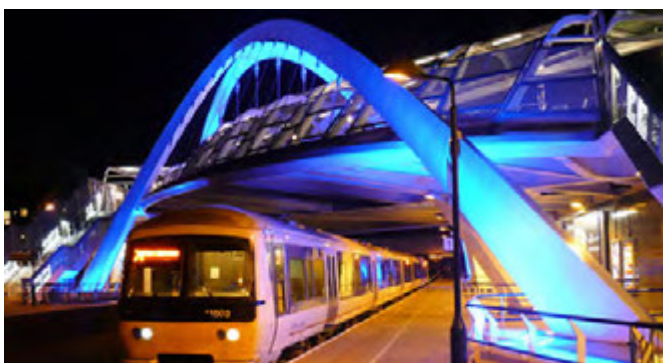
Wembley Station Link - White Horse Bridge
