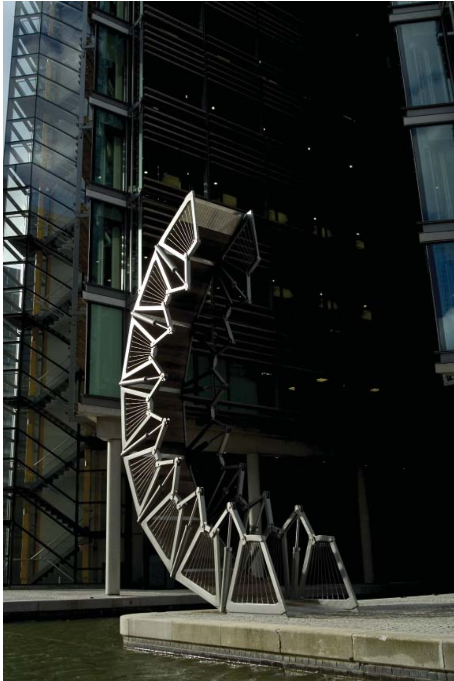
Rolling Bridge, UK
