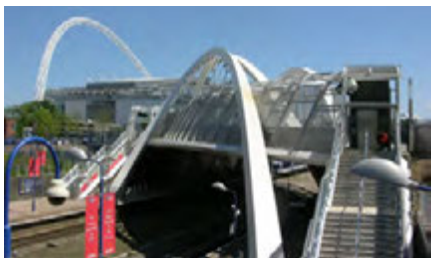
Wembley Station Link - White Horse Bridge
