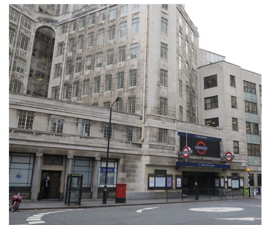
⑦ View of north facade
