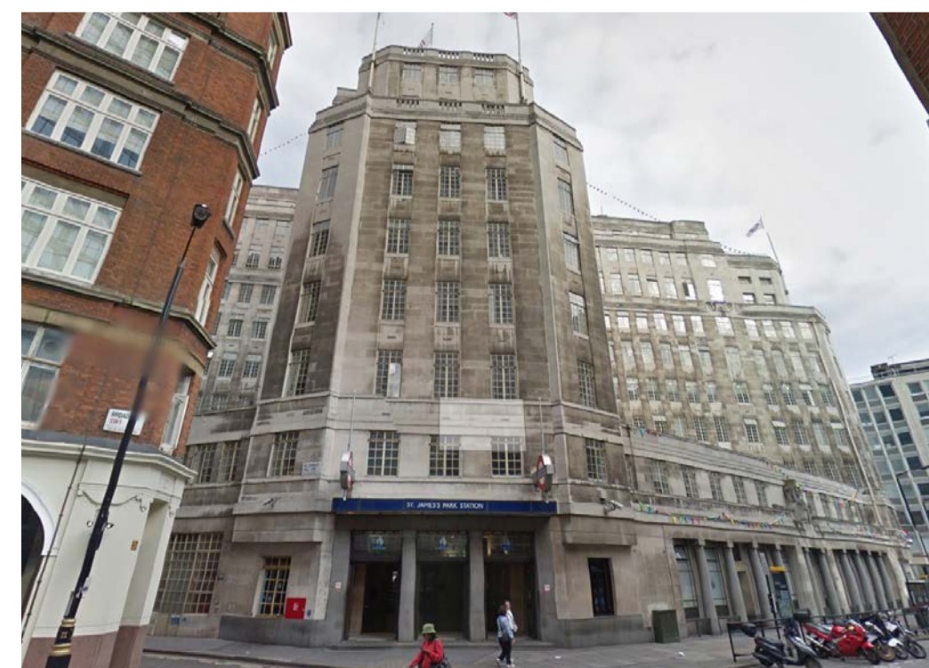
④ South entrance looking down Broadway
