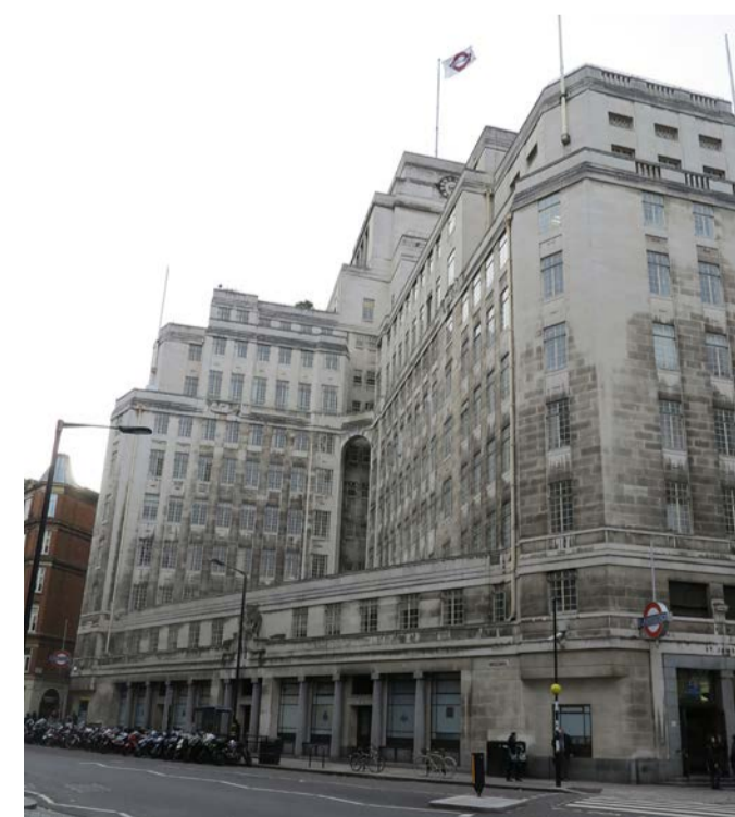
③ View of eastern facade
