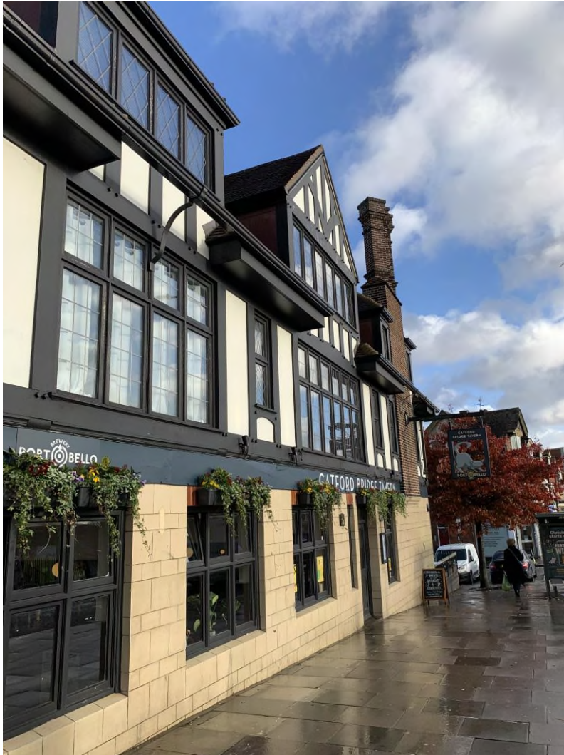
Plate 14: Catford Bridge Tavern, looking east along the pavement of Catford Road
