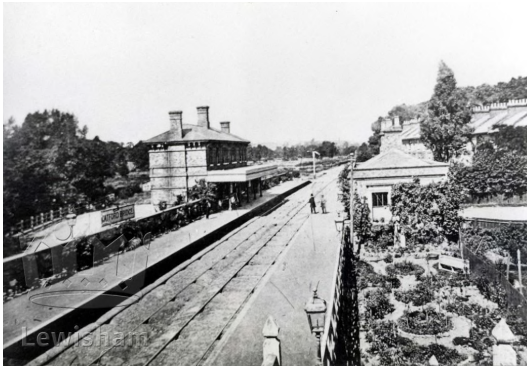
Plate 33: Catford Bridge Station, looking north from Catford Road. Undated. © Lewisham Borough Council
