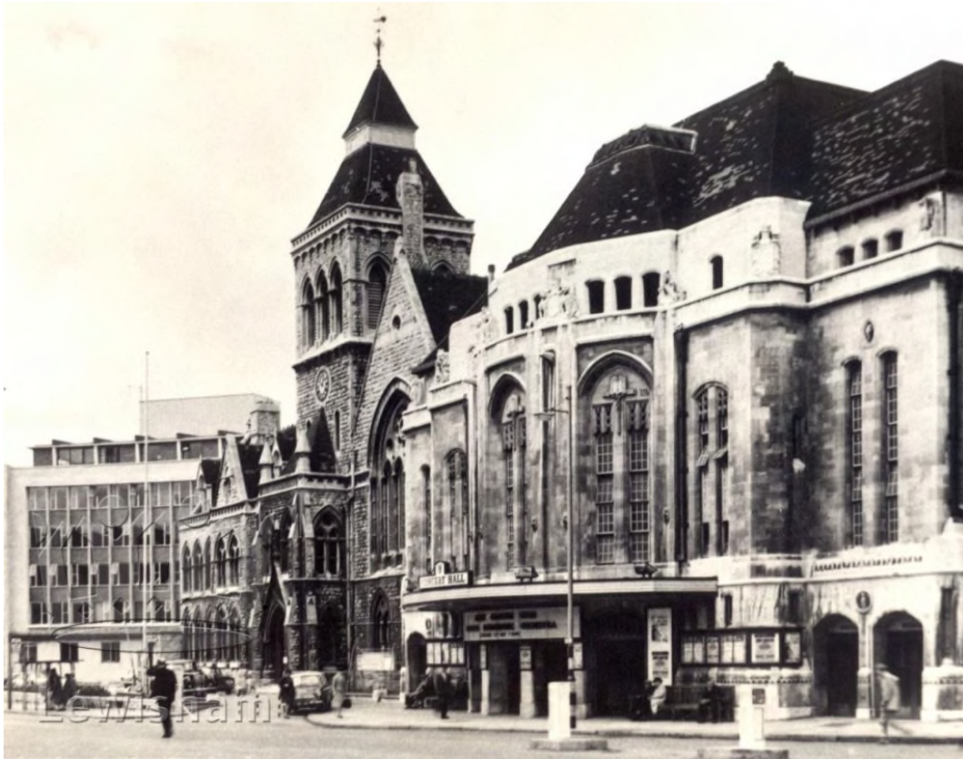
Plate 4: Lewisham Town Hall prior to its demolition in 1968. Flanked to the left by M H Forward's early 1960's council offices and to the right by Lewisham Theatre © Lewisham Borough Photos
