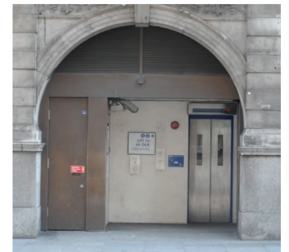
Figure 4.17: Existing entrances to the Bank-Monument Station Complex
