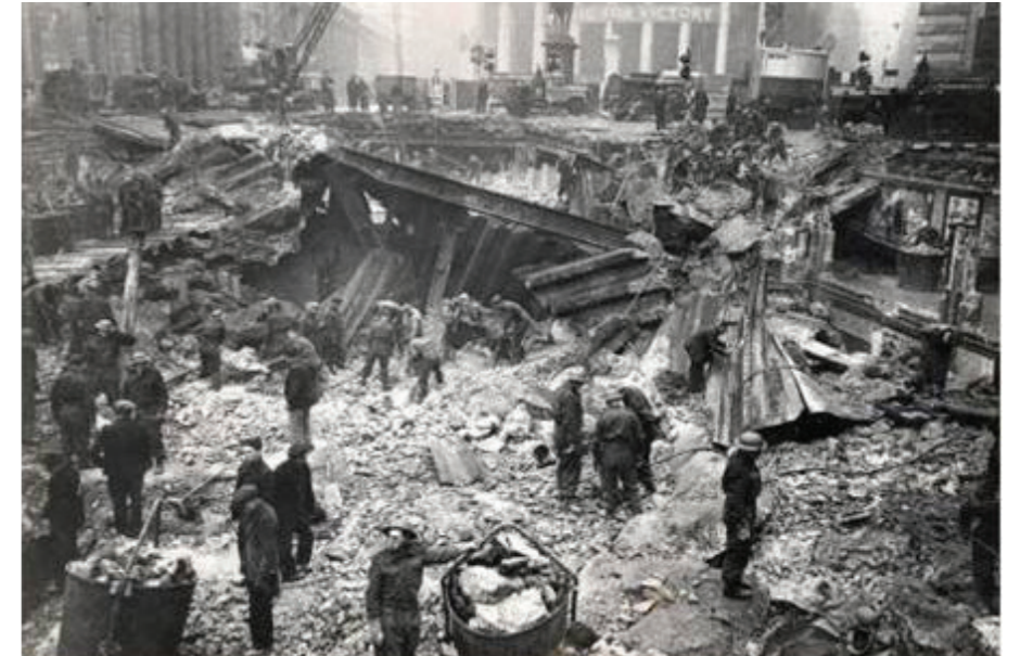
Figure 4.6: World War II bomb damage to Bank Station
