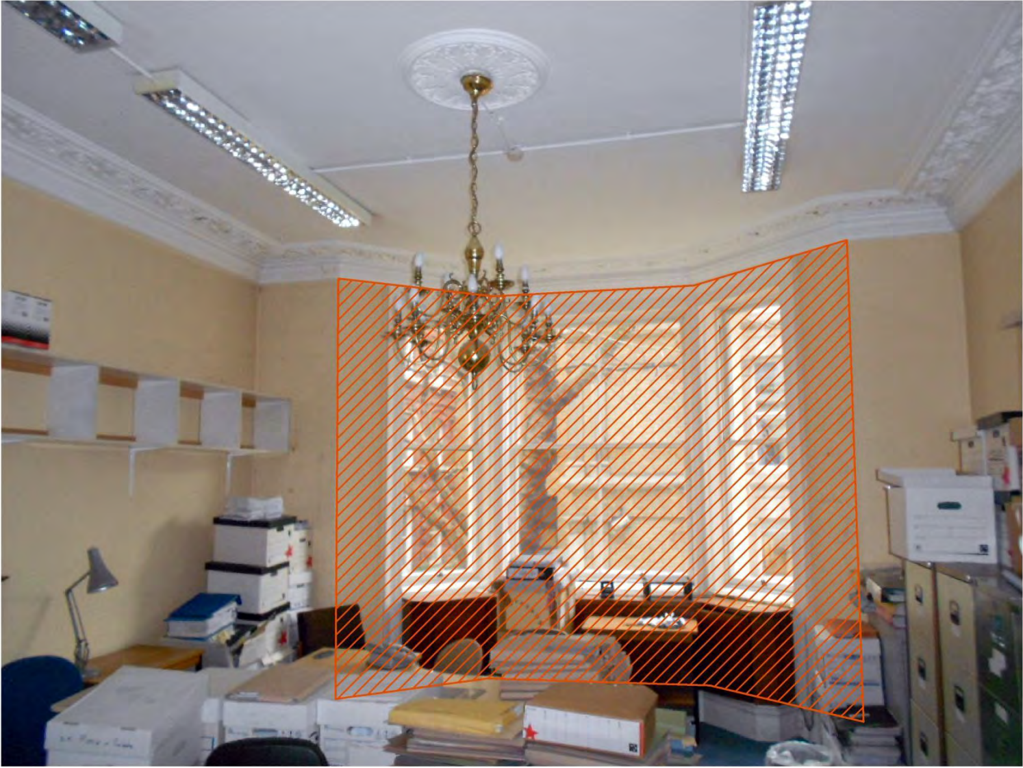
Bay window internal view to the first floor. Note, decorative plasterwork will not be impacted by protective works
