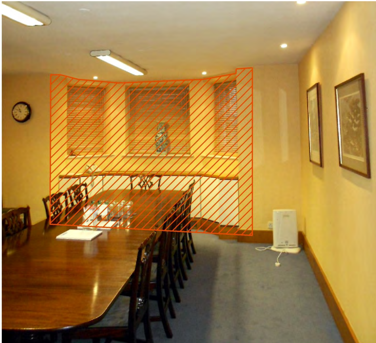
Bay window internal view to the ground floor
