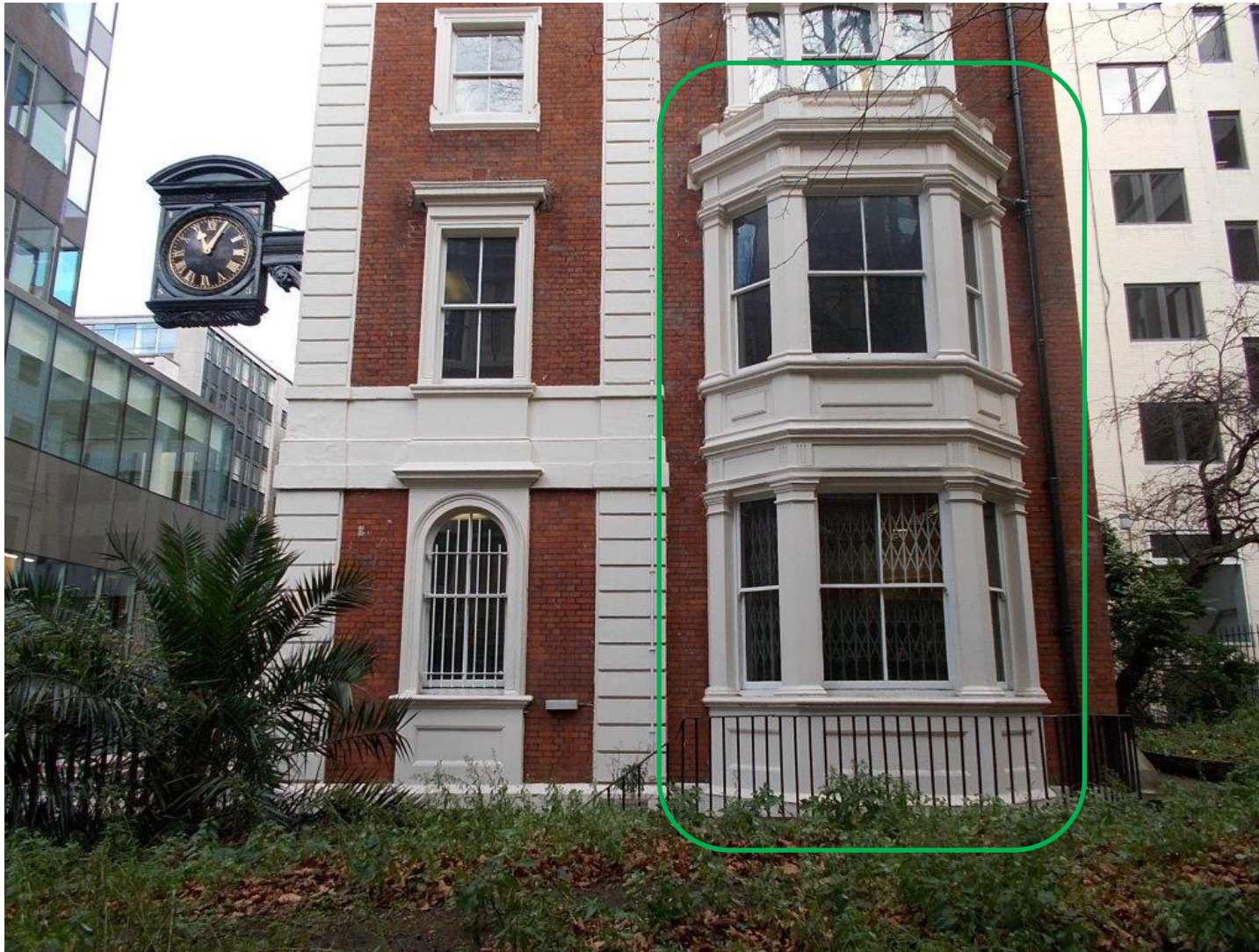
Areas to ground and first floor on south elevation to be impacted by temporary support, with fixings to brickwork
