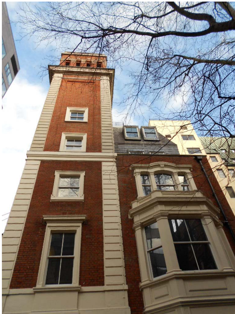
Photo 2: Southern elevation of 29 Martin Lane, tower to left and top of bay window to right
