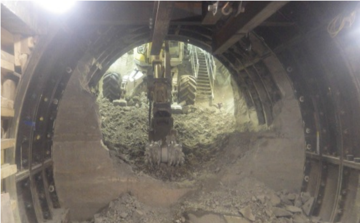
Victoria Station excavation breakthrough into the concourse
