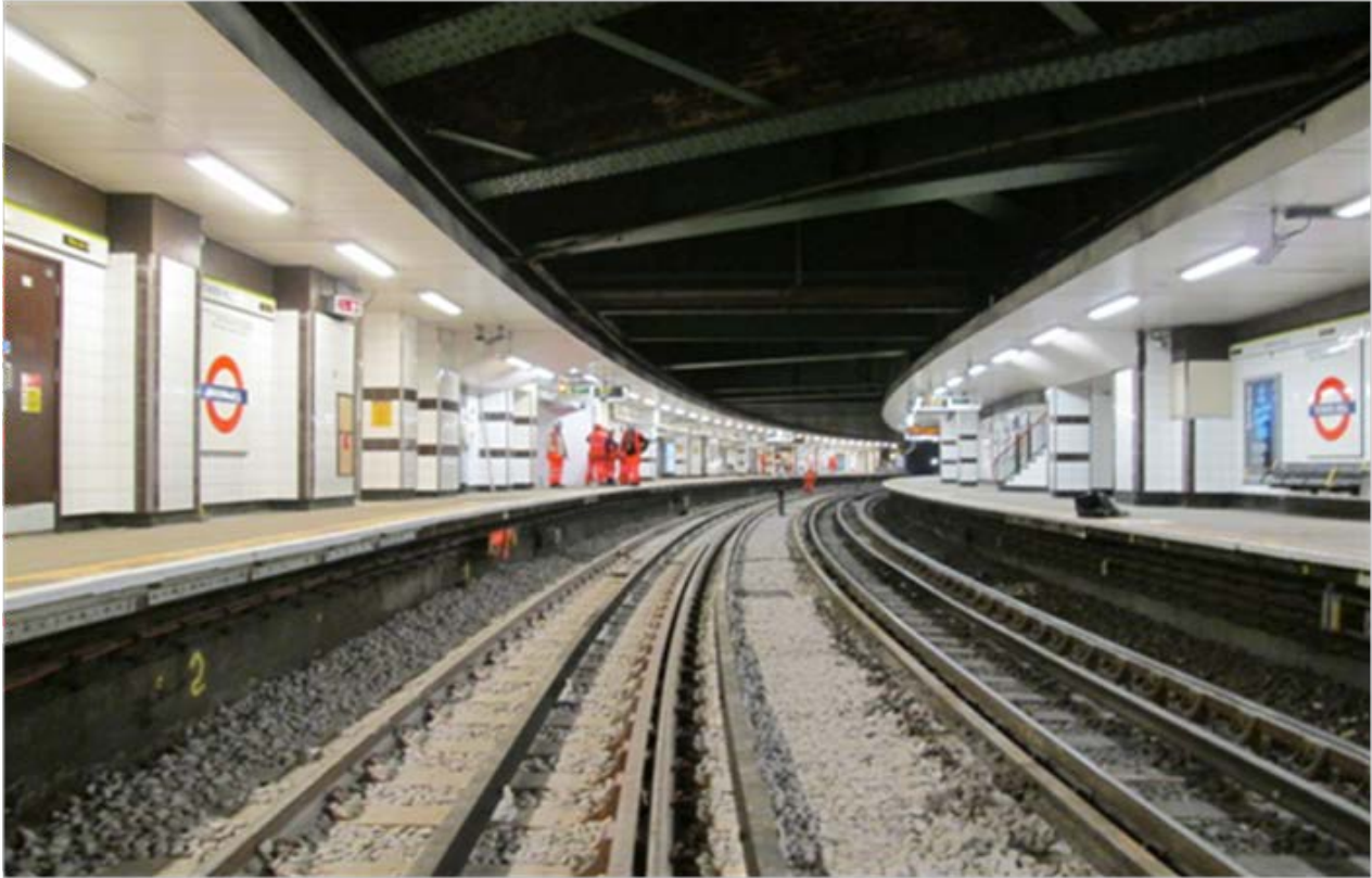
Ballast Track Renewal works at Tower Hill Station
