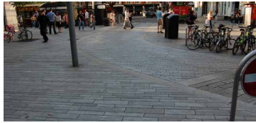
1. Raised and paved carriage way (Granite setts)
