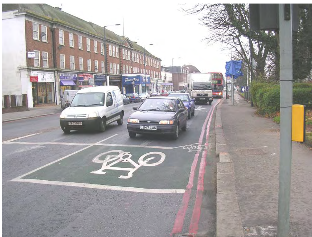
Figure 5.1 – Photo of Site 1
