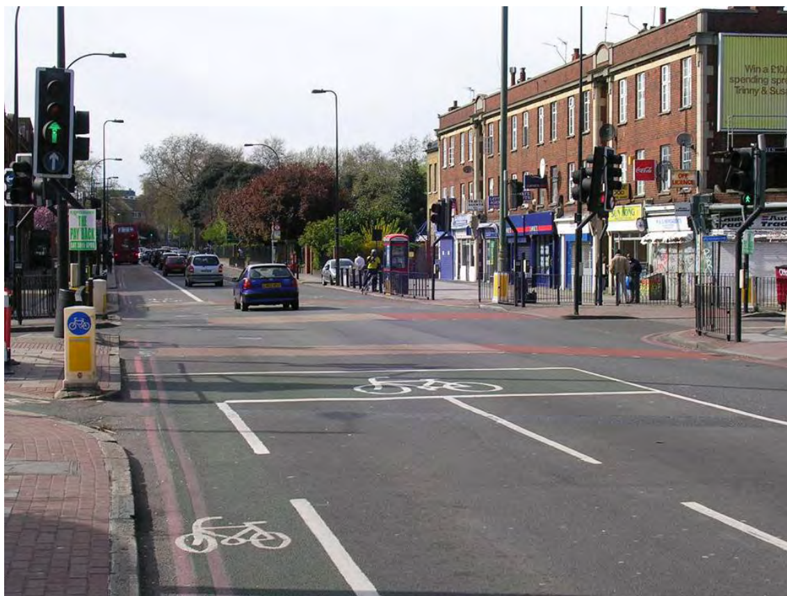
Figure 5.5 – Photo of Site 5
