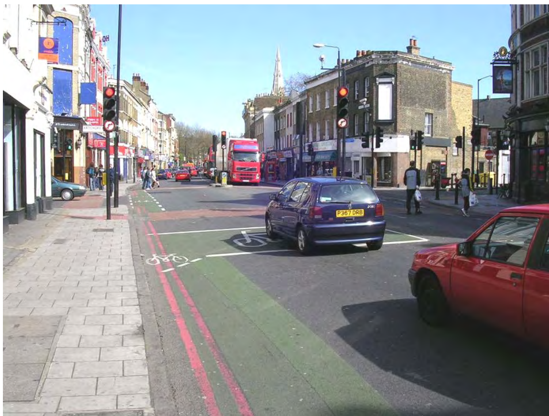
Figure 5.7 – Photo of Site 7
