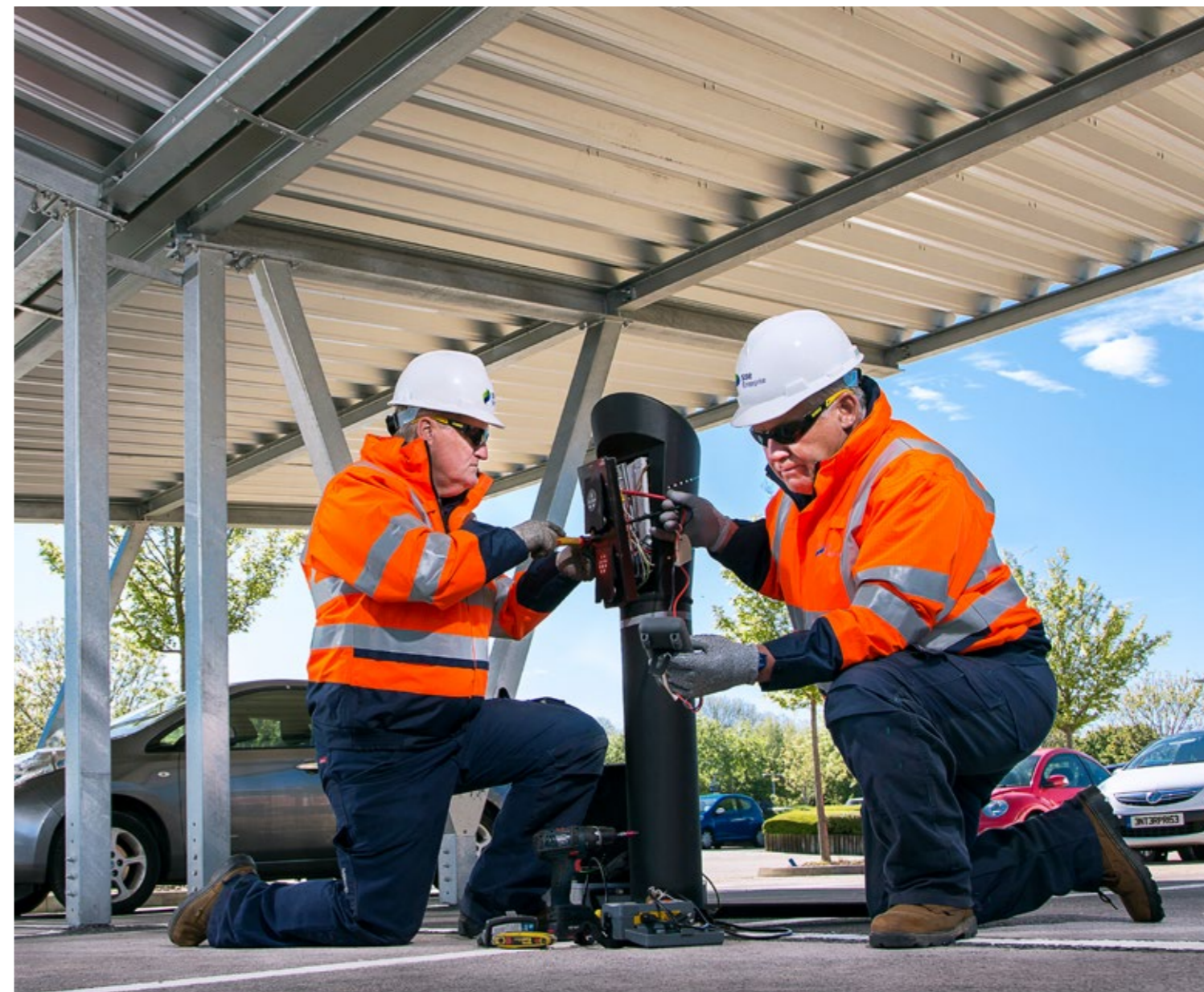
Image 9 Slow charge point being installed in London
