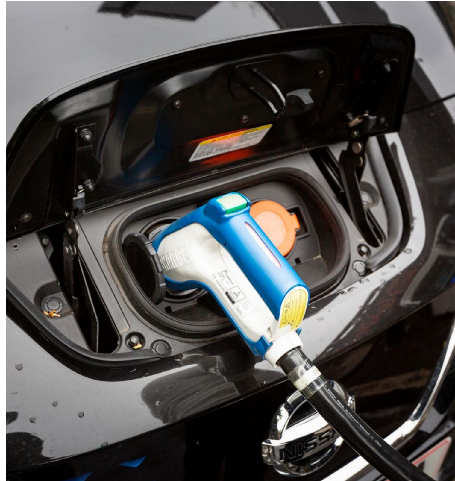
Image 26 EV charge point connector in use
