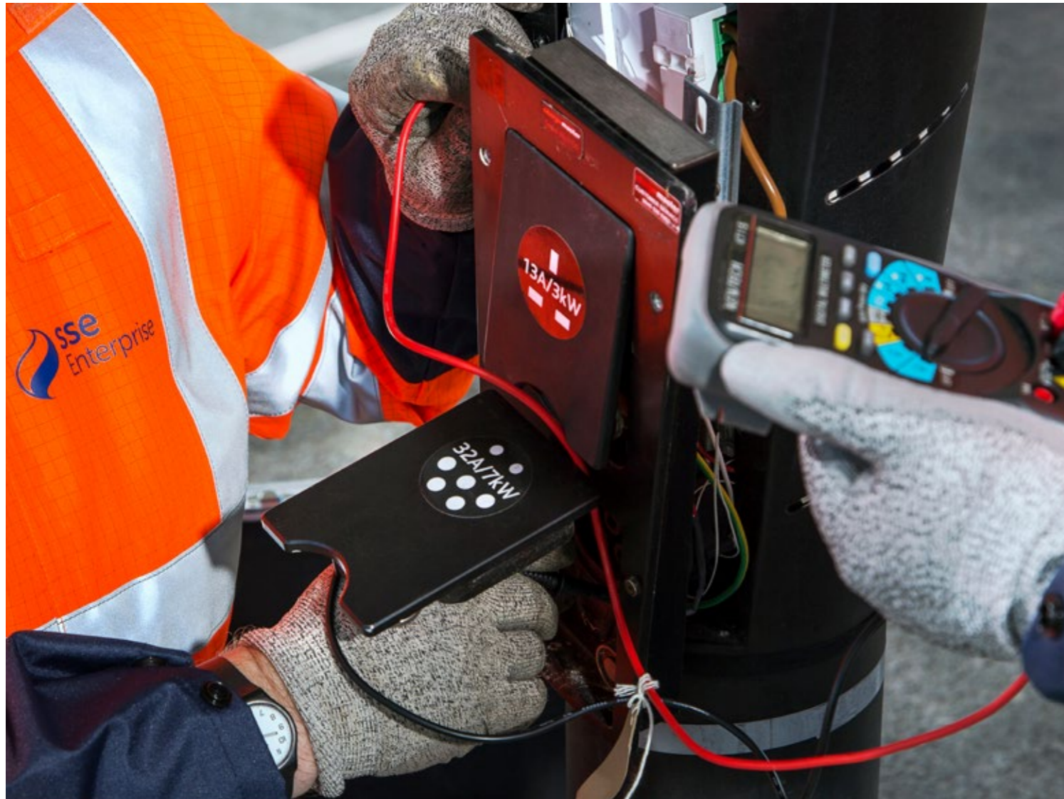
Image 8 Slow charge point being installed in London
