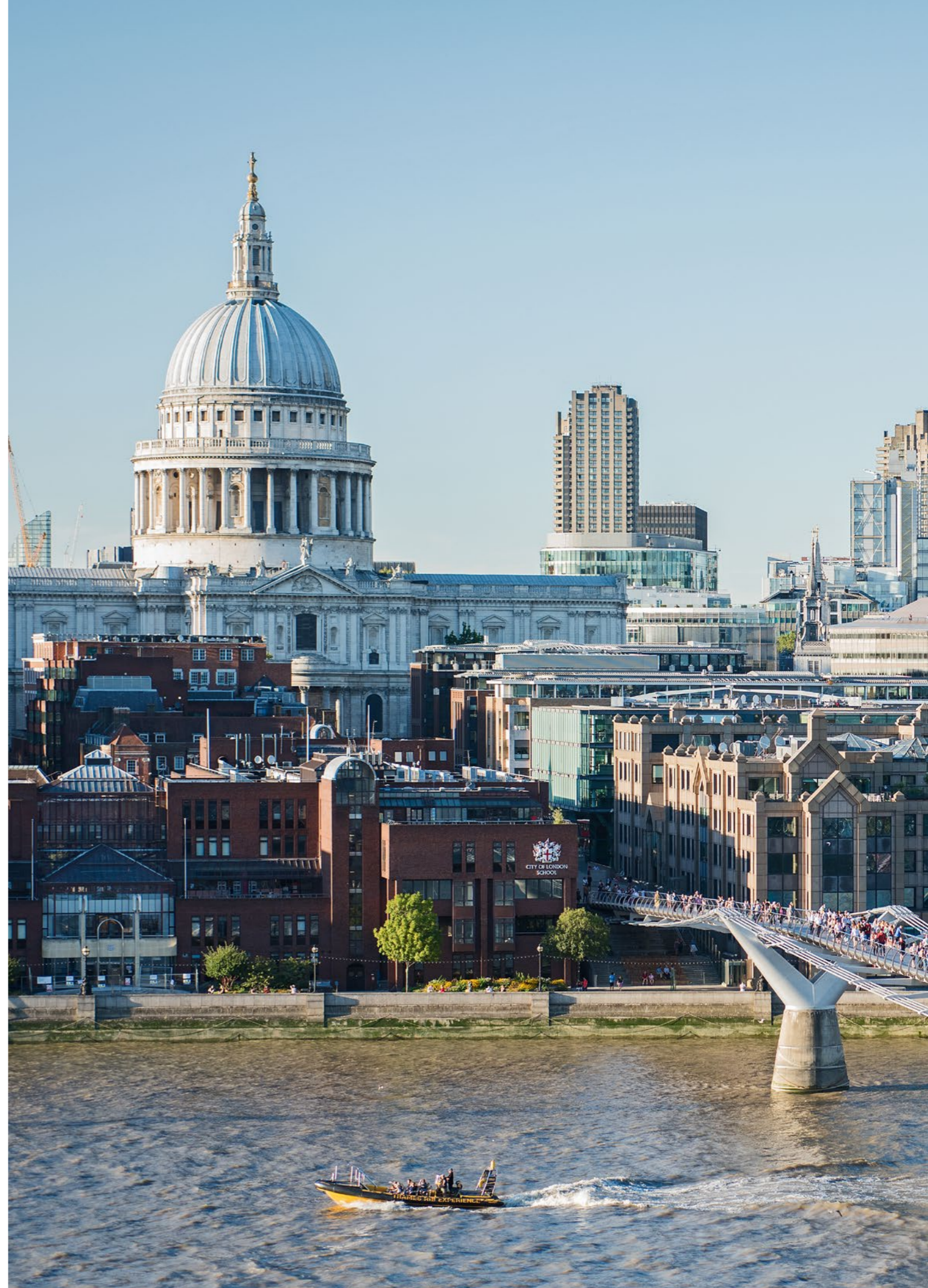
Work is ongoing to address water ingress issues at St Paul's station
