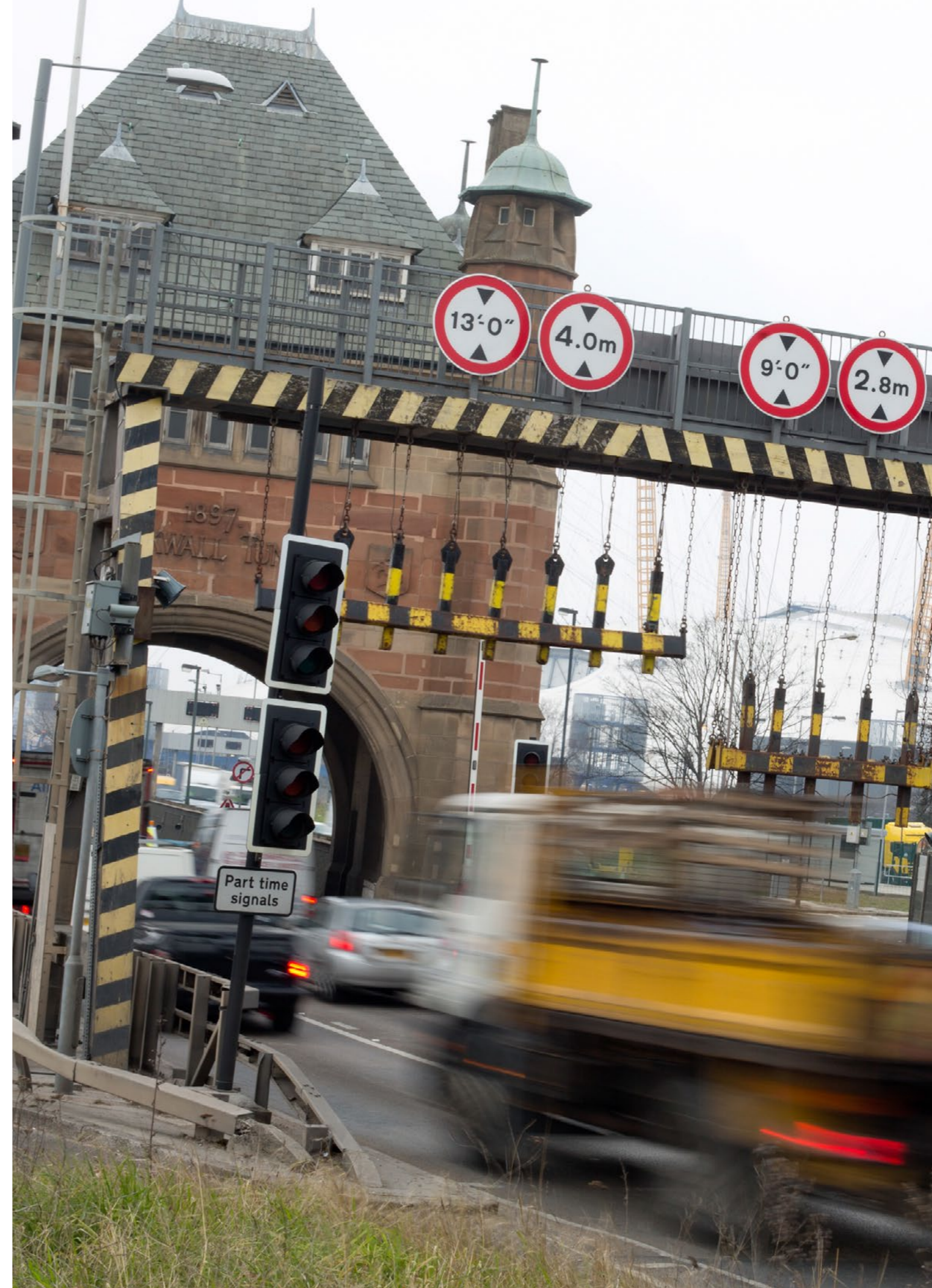
We are renewing critical systems in the Blackwall Tunnel
