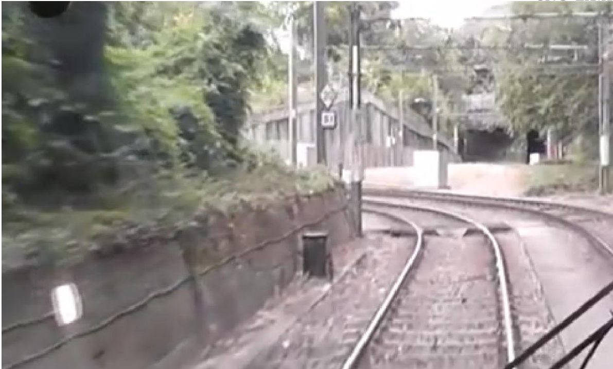
Figure 7 - 20 km/h PSR board on 30m radius curve, with the entrance to the Elmers End/Beckenham Junction branch line showing opposite
