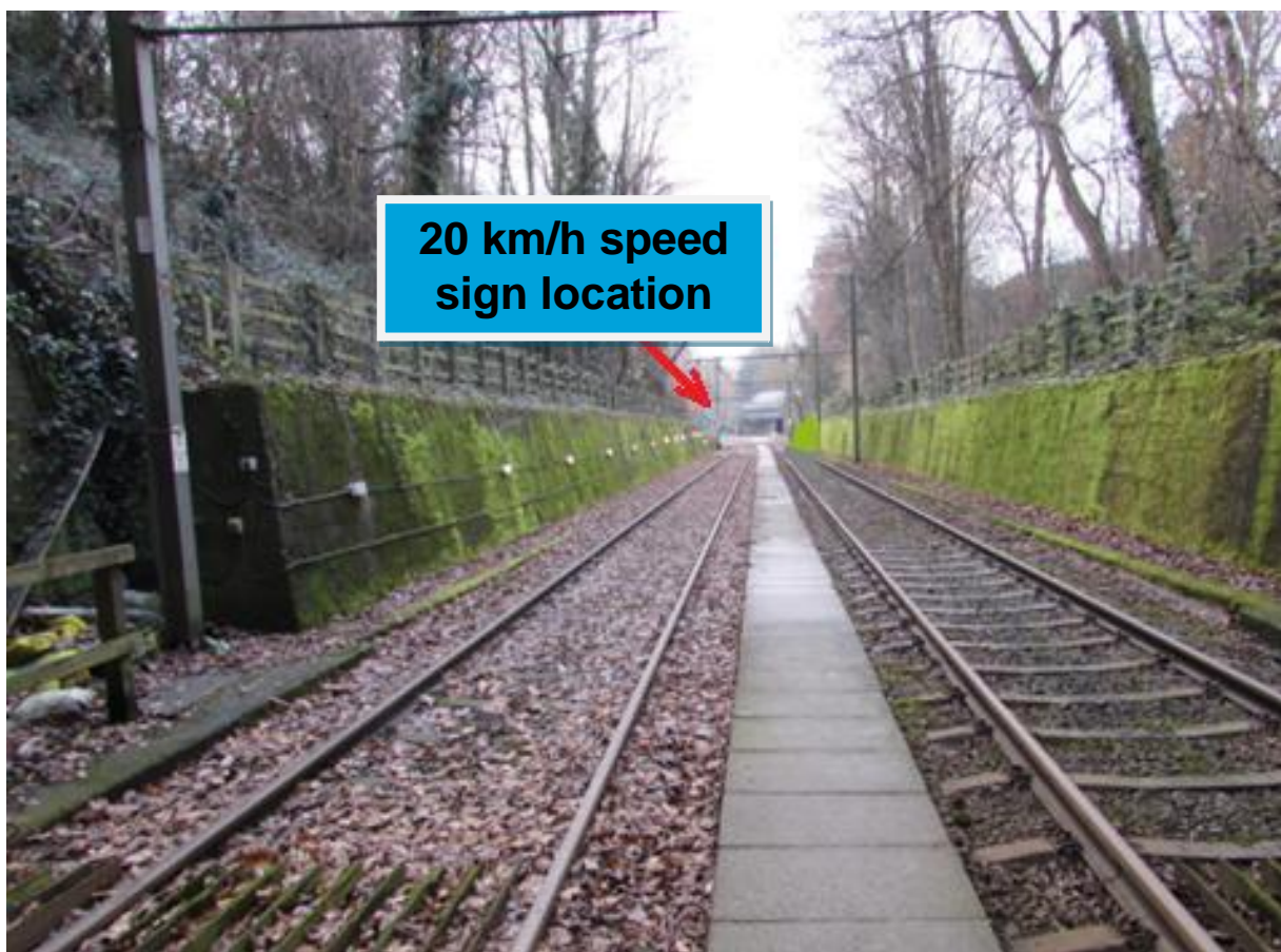
Figure 6 - 20km/h board on exit from Woodside tunnel (photo taken around 85m from the start of the curve)
