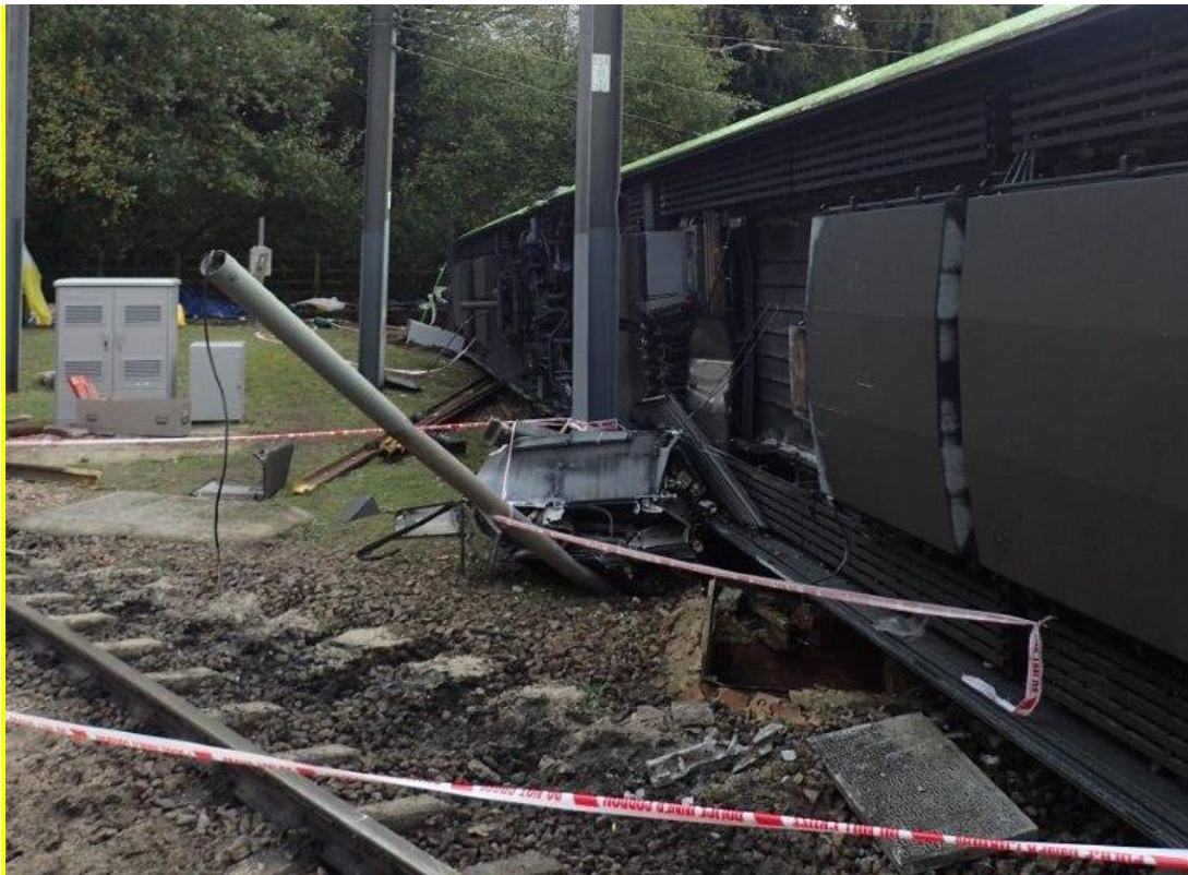
Figure 2 - Tram 2551 roof against infrastructure
