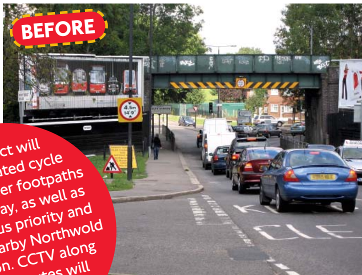
Petts Hill railway bridge is being totally revamped.
