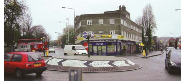
Sydenham's main street, between Cobbs Corner (above) and Mayow Road, is the subject of a street audit.
