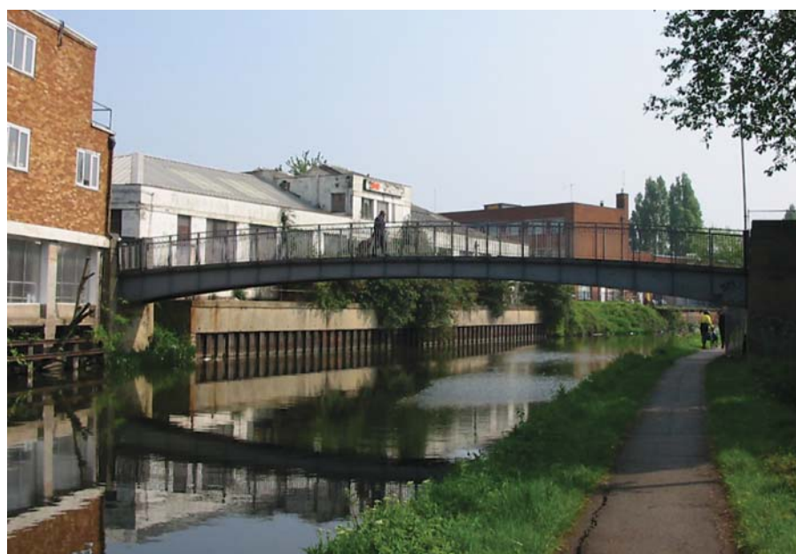
The Carlyon Road footbridge will be upgraded with borough funding.
