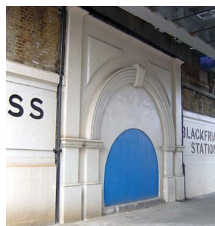
After: the structure has been restored.
