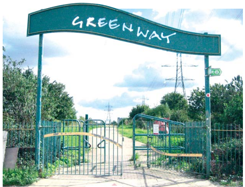
The Elevated Greenway will be improved to maintain an east-west route across the Olympic Park during construction work.
