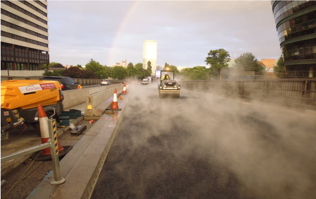
Resurfacing works at Hammersmith Flyover during a weekend closure
