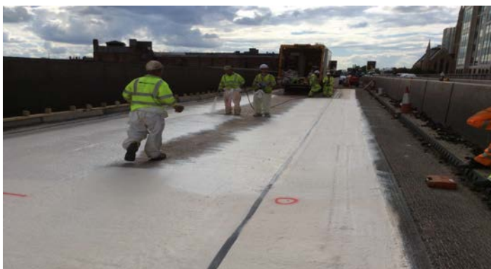
Waterproofing being applied to Hammersmith Flyover during a weekend closure
