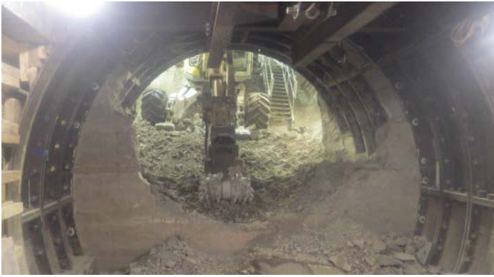
Victoria station excavation breakthrough into the concourse
