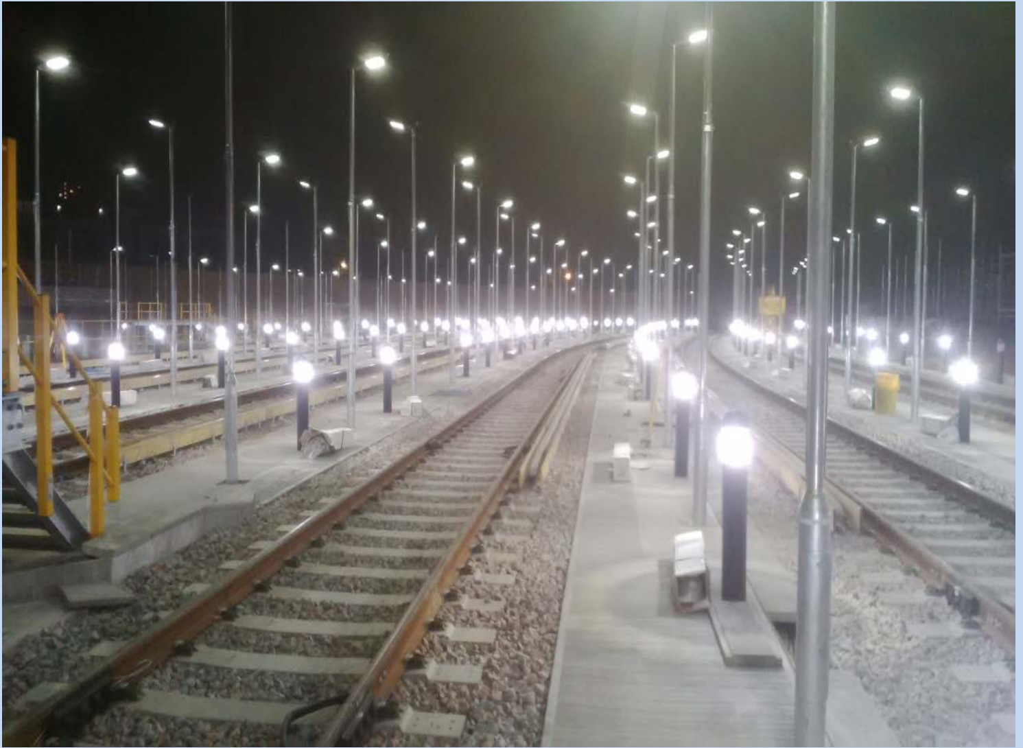
London Rail Stabling Yard Sidings Silwood London Borough of Lewisham
