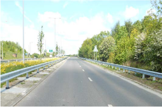
A41 Edgware Way – renewal of 3,046m of vehicle restraint barriers
