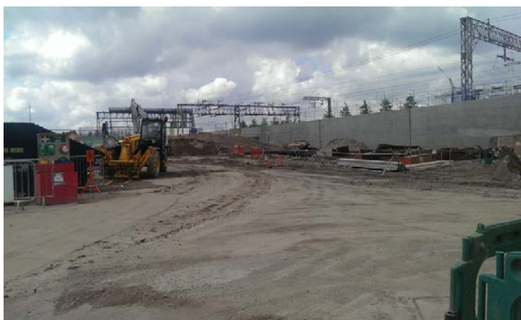
Twin tracking works
