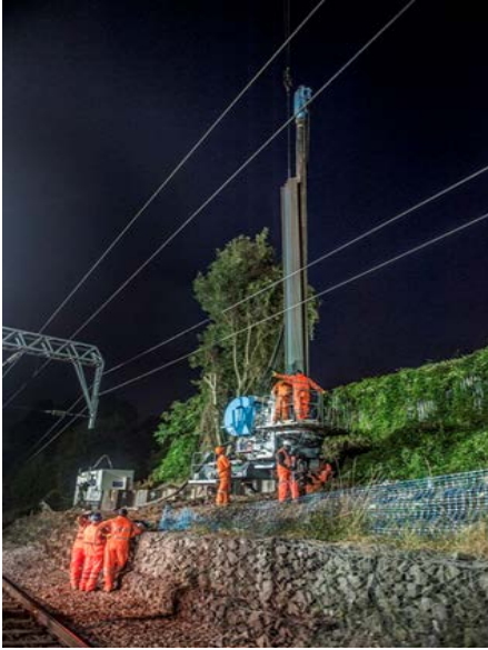
Piling at West Hampstead
