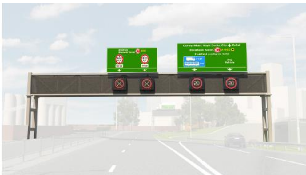
Figure 4-5 Typical gantry and Variable Message Signs (VMS) signs
