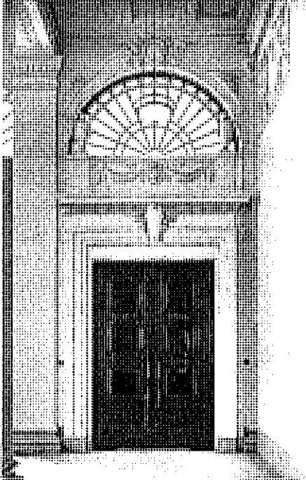
The ENTRANCE DOORS .—The doors are in oak and bronze and the fanlight is bronze.
