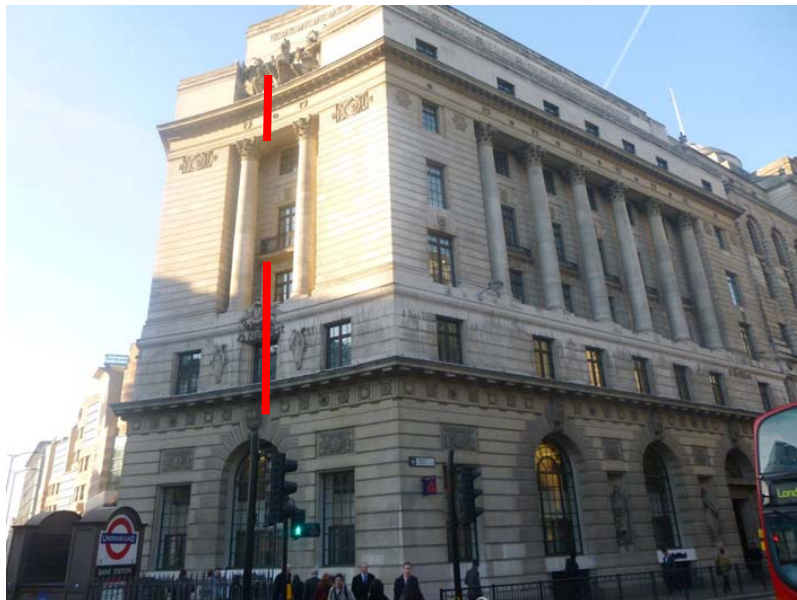
Photo 2: Predicted concentration of strains to 1 Princes Street elevation
