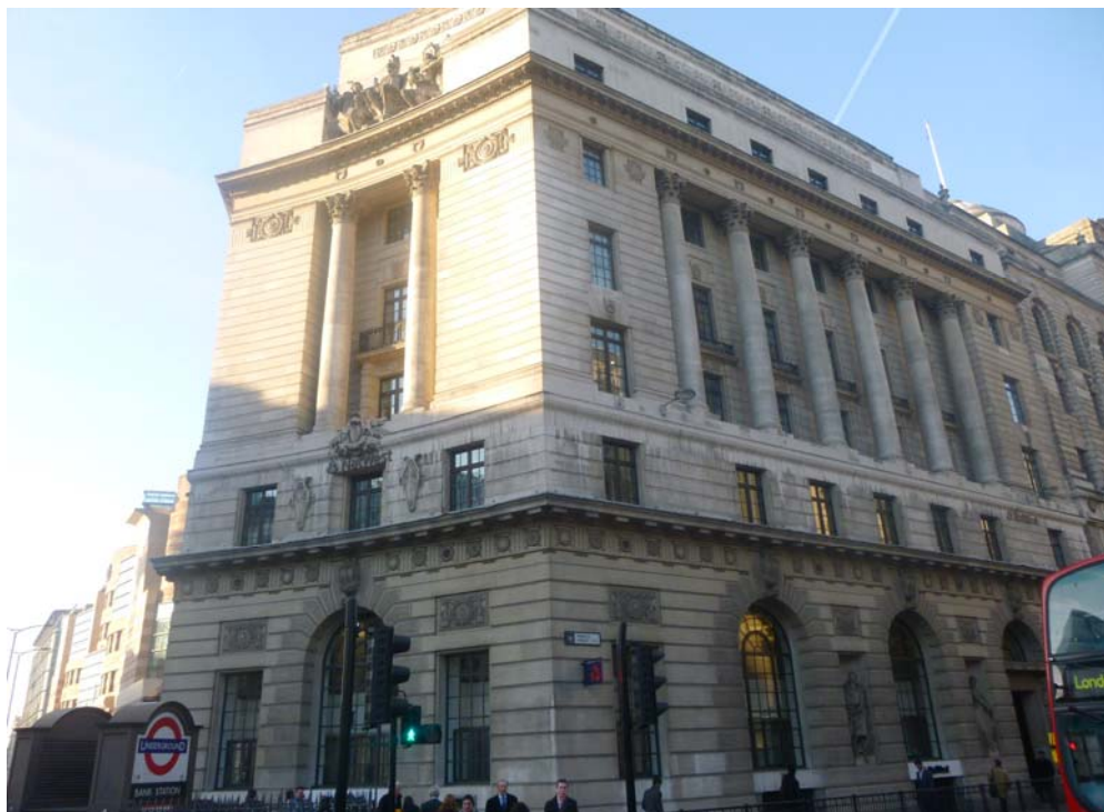
Photo 1: General view of 1 Princes Street
