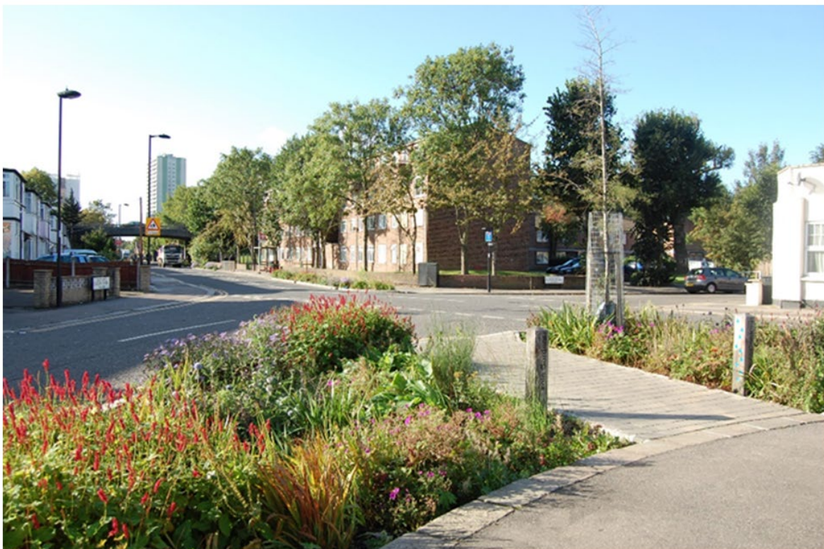
Figure 13. SuDS rain garden incorporated in a kerb build-out in London Borough of Enfield.
