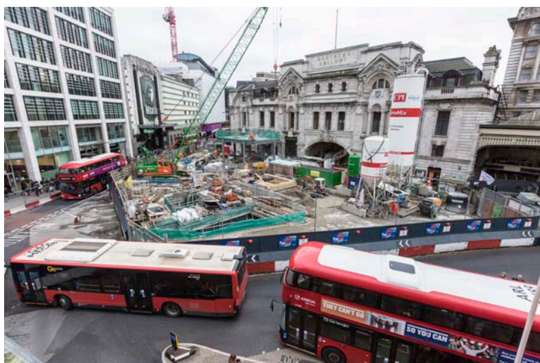
Works in progress outside the main entrance to Victoria railway station
