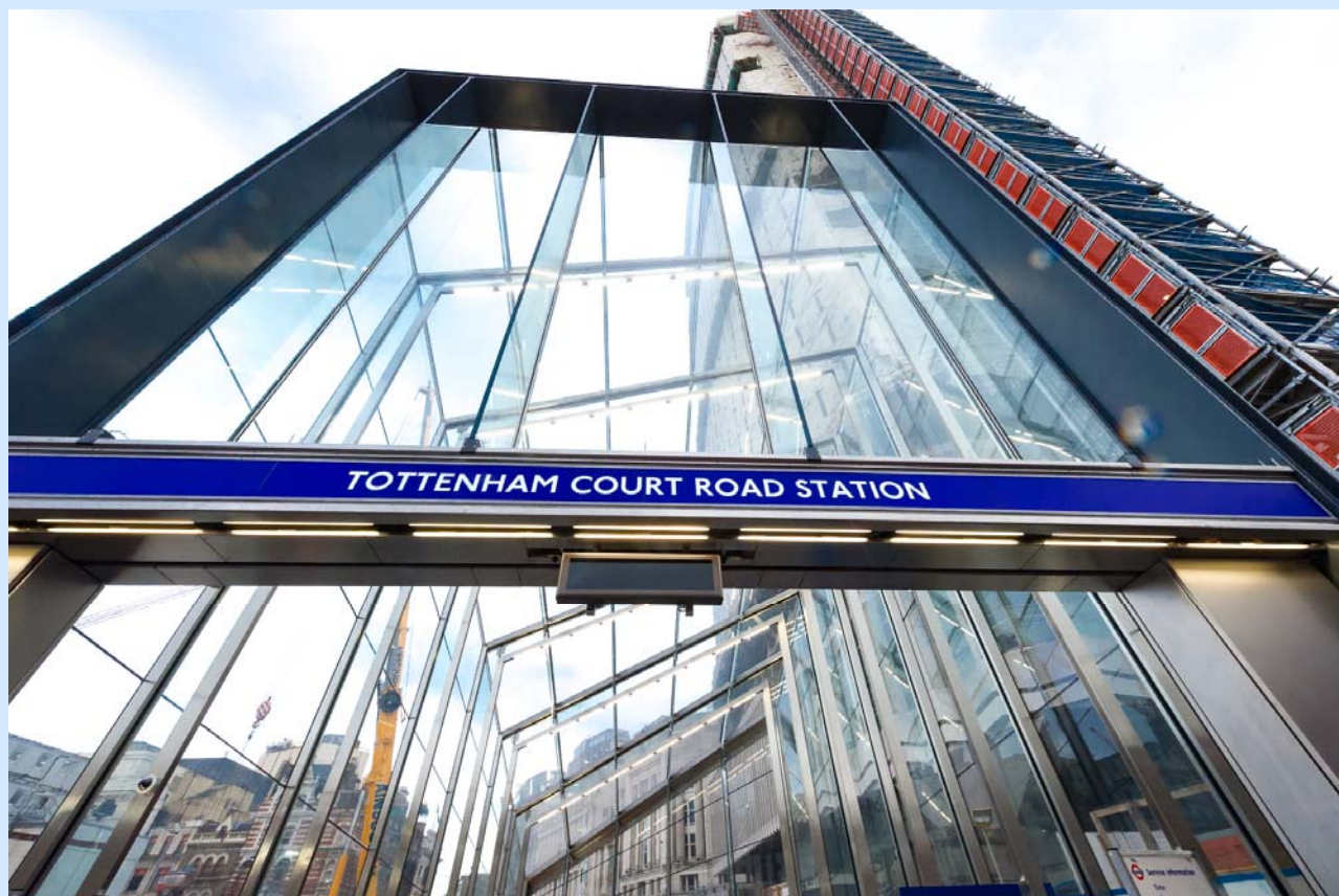
The new south plaza entrance
