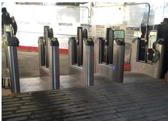
New gateline at South Tottenham station
