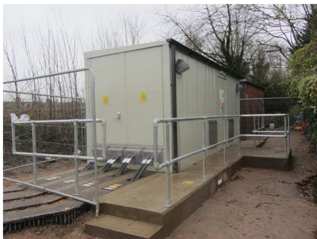
The track paralleling hut at Southfields
