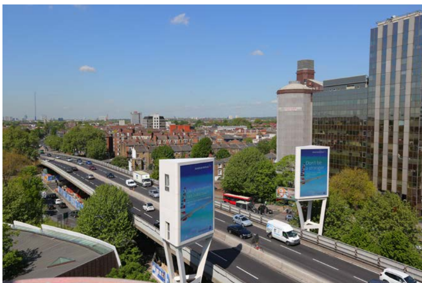
The Hammersmith Flyover
