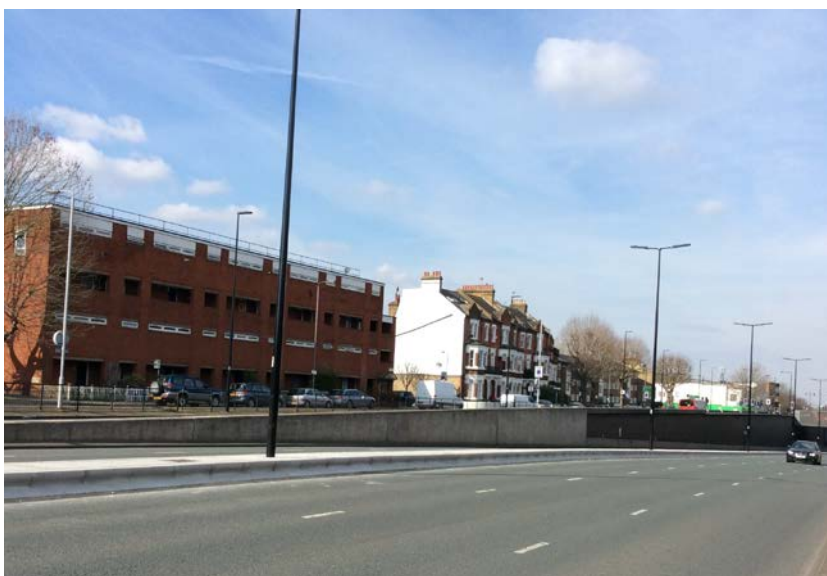
Replaced lighting luminaires and columns in Trinity Road
