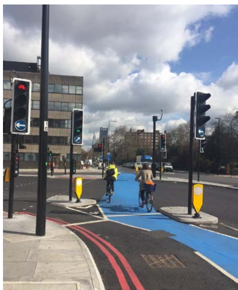
Cycle facilities are fully operational at Oval
