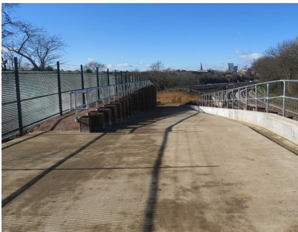
Hanger Lane RRAP Phase I works completed
