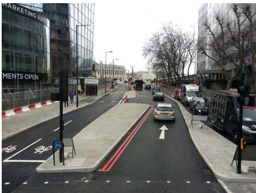
Blackfriars Road following resurfacing
