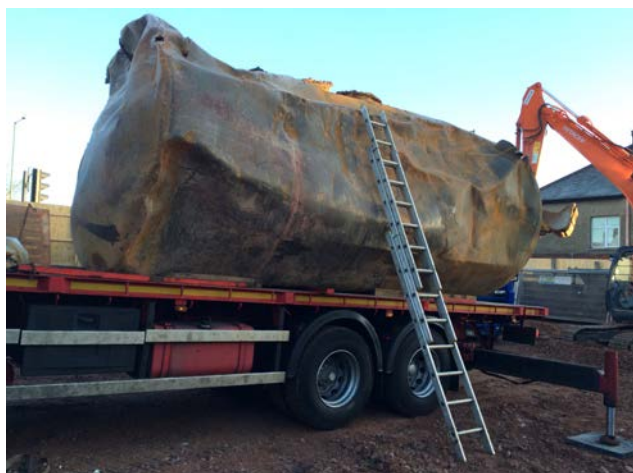
Removal of one of four redundant fuel tanks and construction activities in progress at the Brentfield Road scheme
