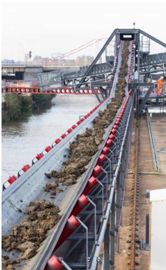
The muck-away conveyor
