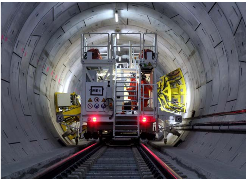
Crossrail's innovative automated drilling machine
