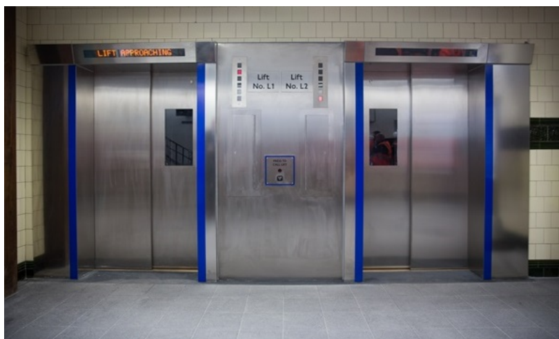
The new lifts at Tufnell Park station
