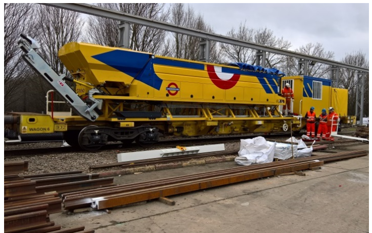
Concrete mixer mounted on donor wagon
