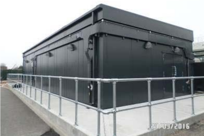
Hammersmith signal equipment room, which has been completed and handed over to Thales to start installation of the ATC signalling system
