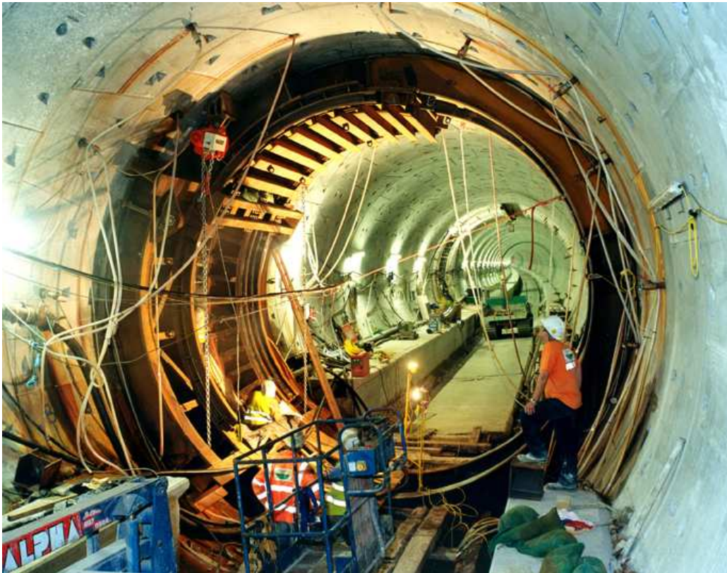
Cross Passage Construction CTRL C320
