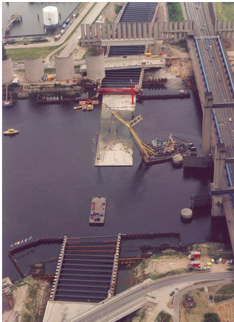
Typical cofferdams at river wall for an immersed tunnel
