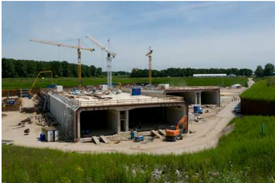
Typical earthworks casting basin (Barrendrecht, Netherlands)
