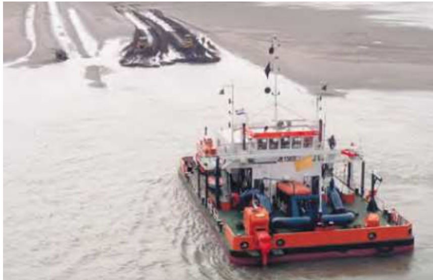
WID dredger for maintenance
