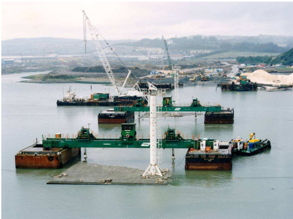
Tunnel element being warped across the River Medway ready for immersion
