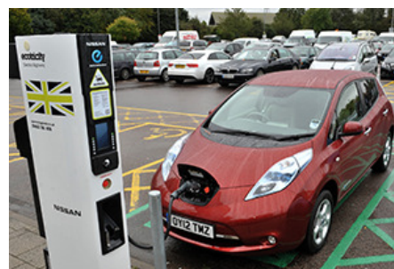
Figure 9 – A charge point of the Electric Highway
