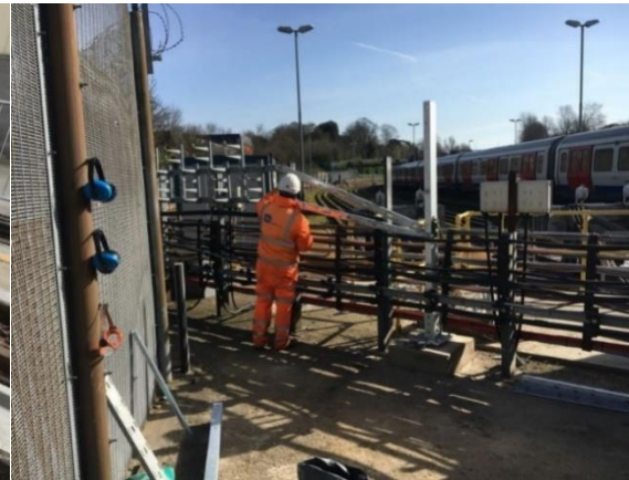
Figure 4 – Cable Route installation at Uxbridge
