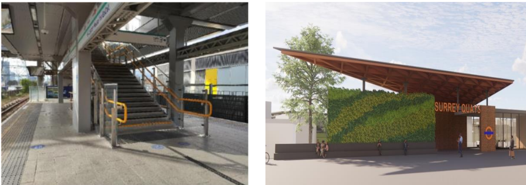
Figure 2: Stairs to new mezzanine level at Custom House station (left) and impression of the new accessible entrance at Surrey Quays station (right)
