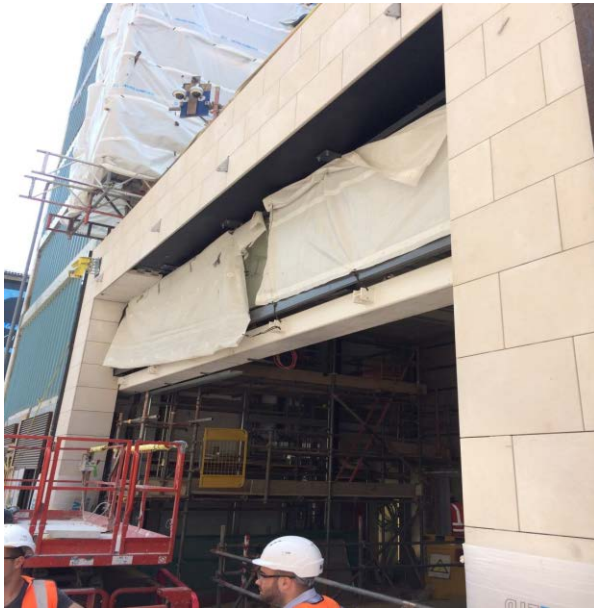
Figure 2 Construction of new entrance on Marylebone Lane
