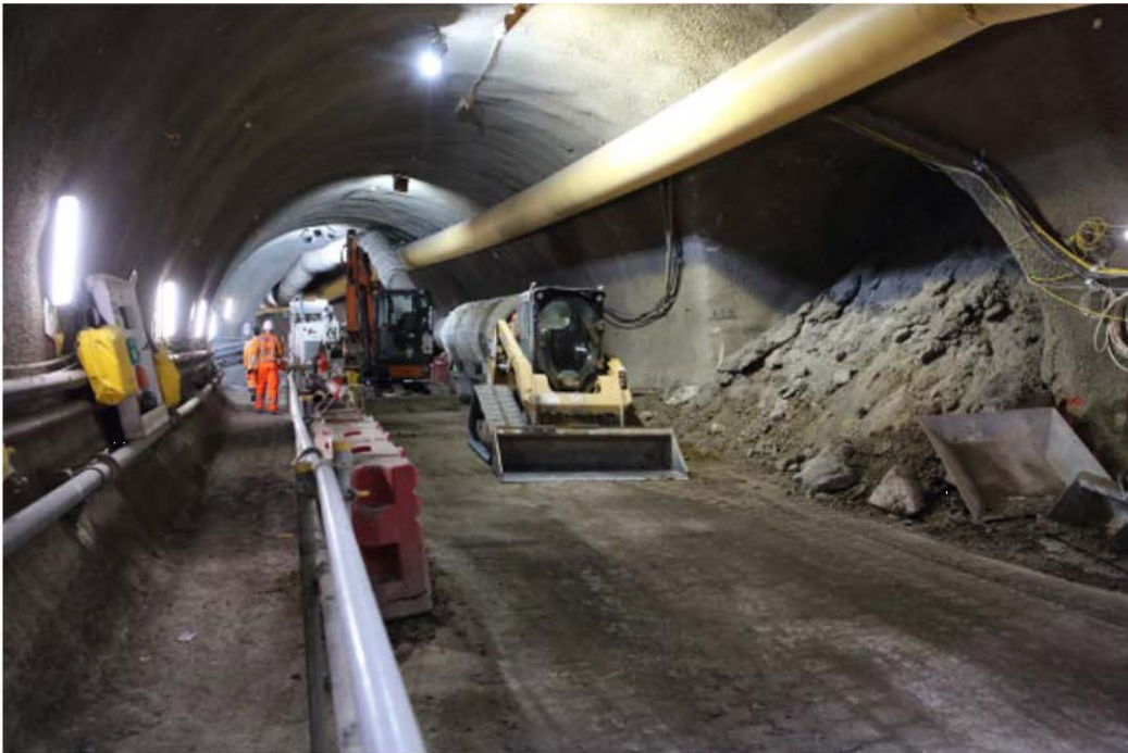
Figure 3 Progress photo: Tunnelling the new southbound Northern line
