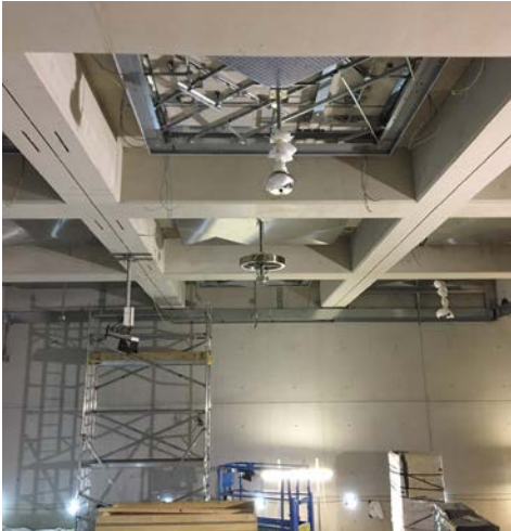
Figure 2 - Installation of ceiling at intermediate level
