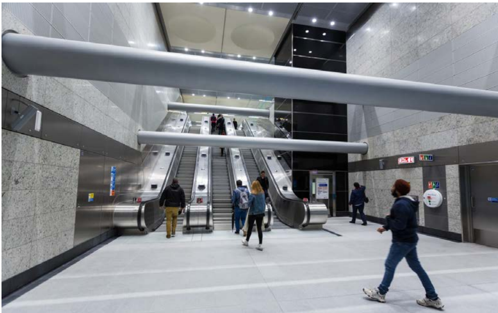
Figure 3: Escalators and lift leading to New Bressenden Place North ticket hall
