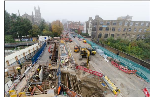
Upper Holloway - replace the deck of the road-over-rail bridge
