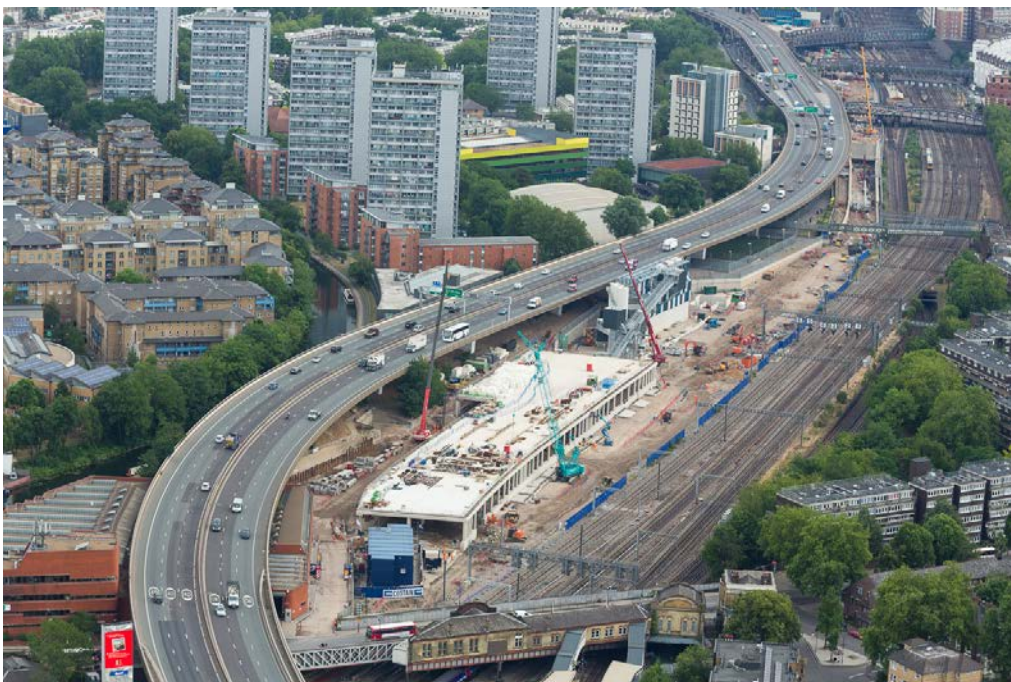
Section 5, looking eastwards from Westbourne Park Station
