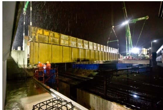
Ardleigh Green - replace the entire road-over-rail bridge
