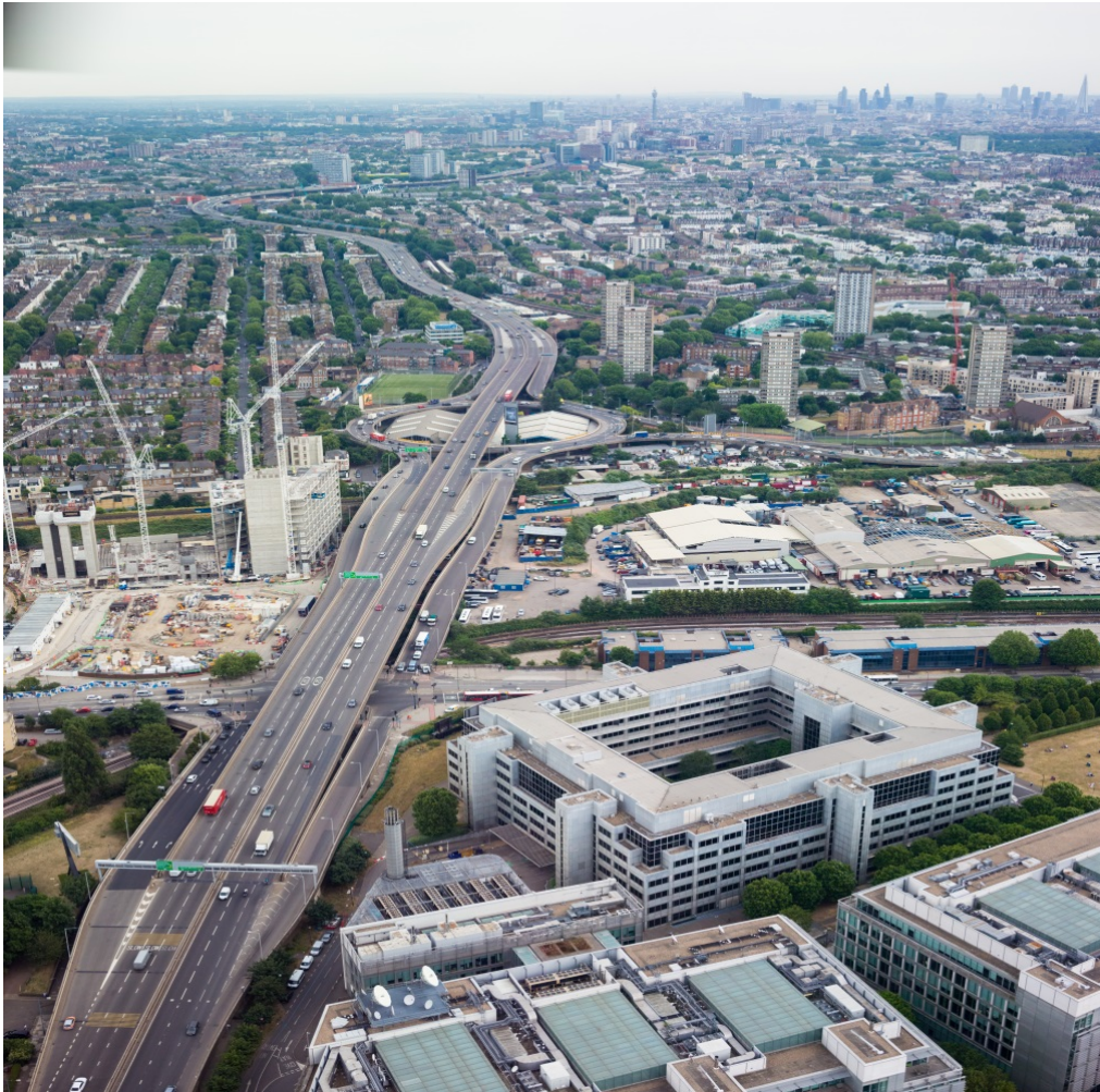
Wood Lane Flyover and the Elevated Roundabout
