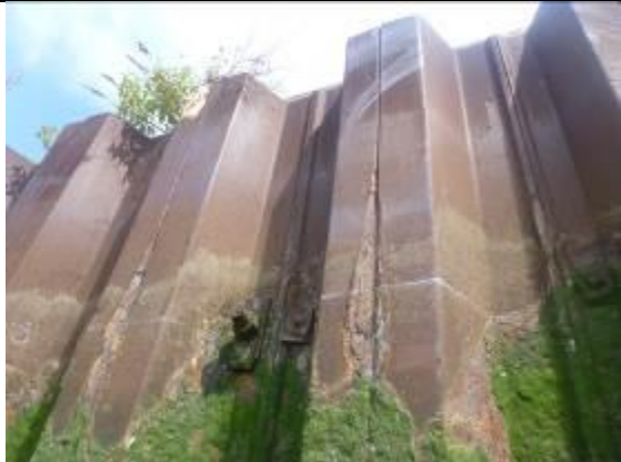
Figure 33 - Waling bolt on sheet pile wall
