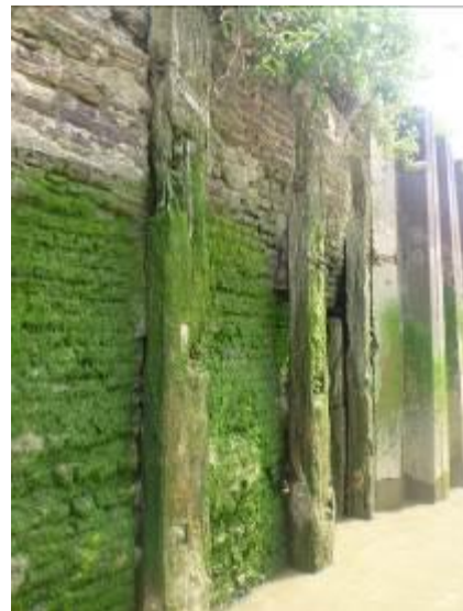
Figure 32 – View of algal growth and remains of timber fenders at downstream extent of asset
