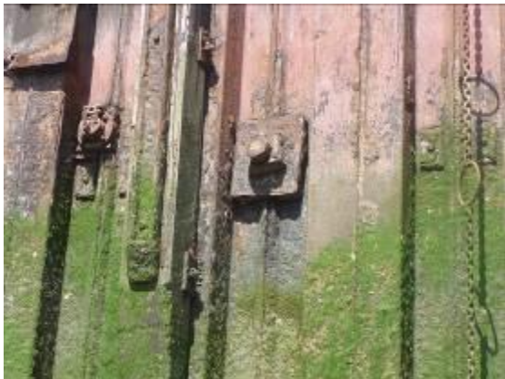
Figure 72 - Corroded waling and anchor bolts
