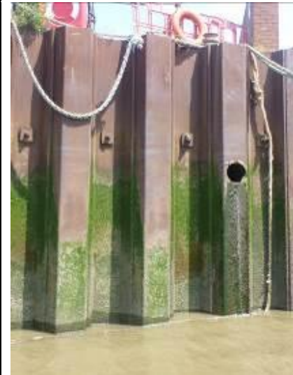
Figure 46 - Hole in sheet piling indicating missing flap valve
