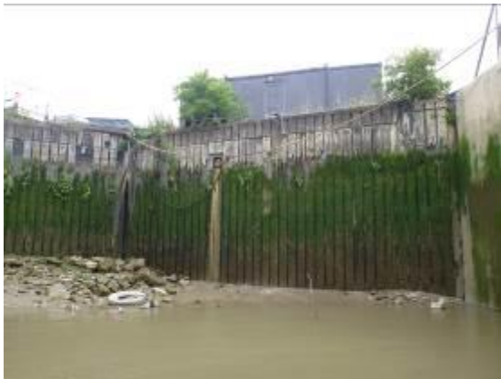
Figure 55 - Steel lock gates with close centred timber cladding
