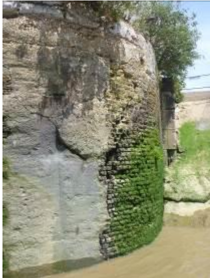
Figure 22 - Large vertical crack in masonry section
