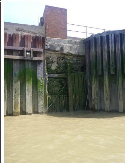
Figure 71 - Steel sheet pile walls with waling and anchor bolts
