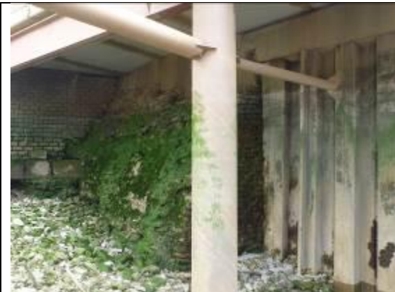
Figure 5 - Concrete bagwork section with steel frame for spoil transfer hopper in foreground
