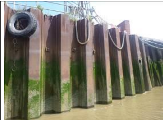
Figure 44 – Pile non-verticality
