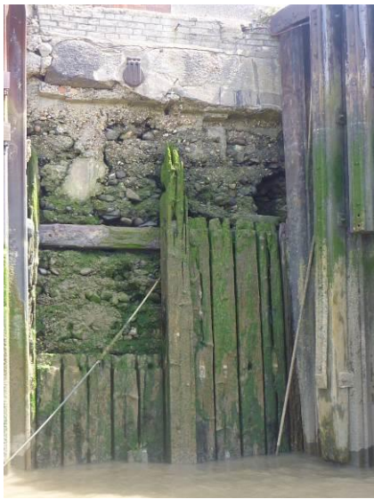
Figure 72 - Corroded waling and anchor bolts
