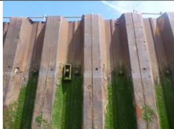
Figure 41 - Waling and anchor bolts
