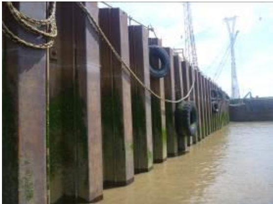
Figure 47 - Steel sheet pile wall
