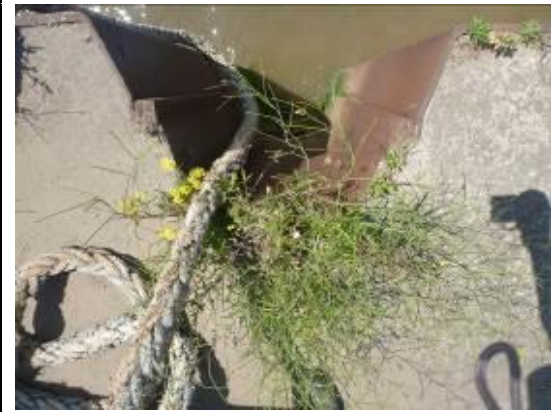
Figure 46 - Hole in sheet piling indicating missing flap valve
