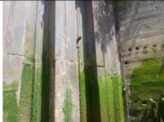
Figure 62 - Section of sheet piles which have been horizontally spliced
