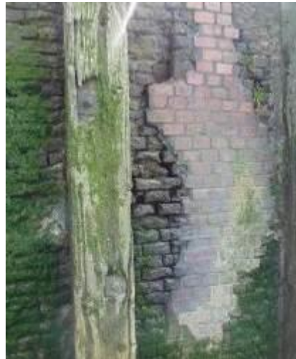
Figure 27 - Repaired section of masonry wall
