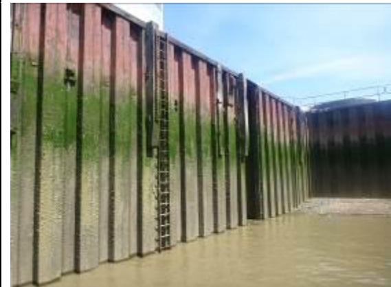
Figure 71 - Steel sheet pile walls with waling and anchor bolts
