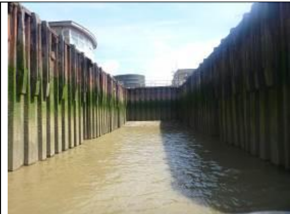
Figure 69 - Steel sheet pile dock
