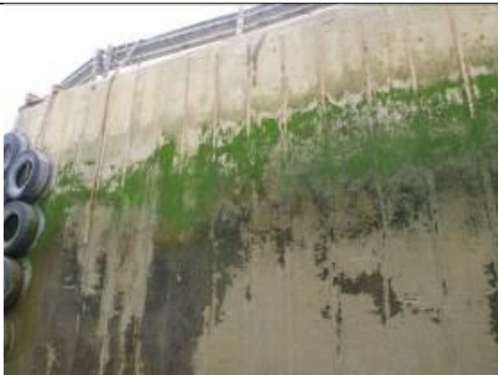
Figure 53 - Concrete abutments with steel railing reinforcement
