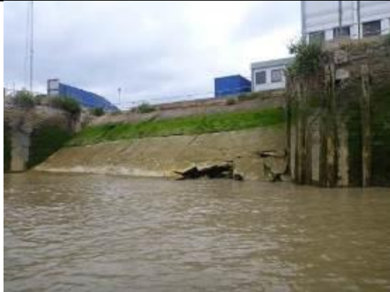
Figure 24 - Concrete apron and masonry abutments
