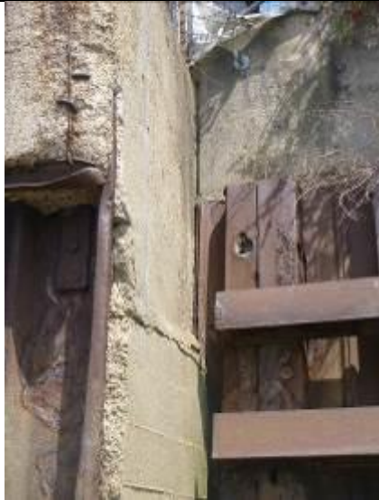
Figure 63 - Interface between steel sheet pile wall and adjacent upstream asset
