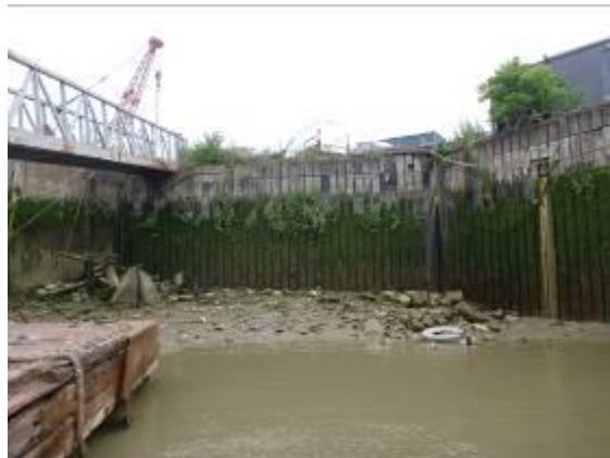
Figure 54 - Steel lock gates with close centred timber cladding
