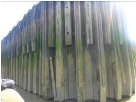
Figure 70 - Timber fenders on entrance to the dock
