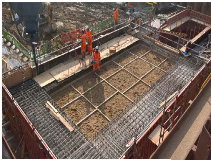
Capping beam construction
