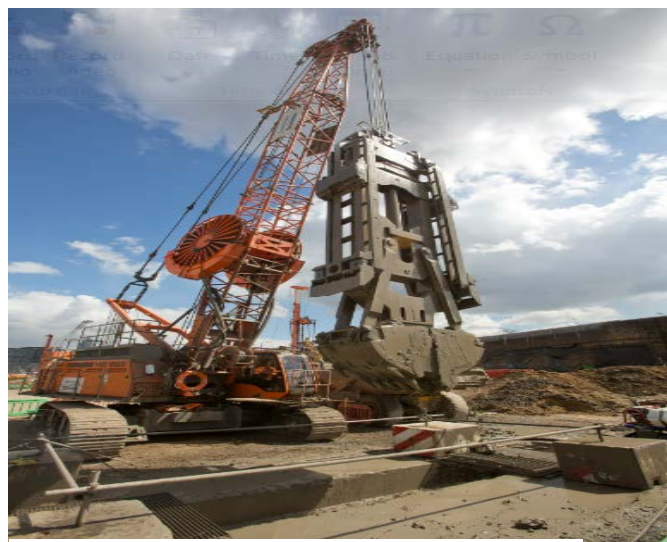
Diaphragm wall construction in the station box
