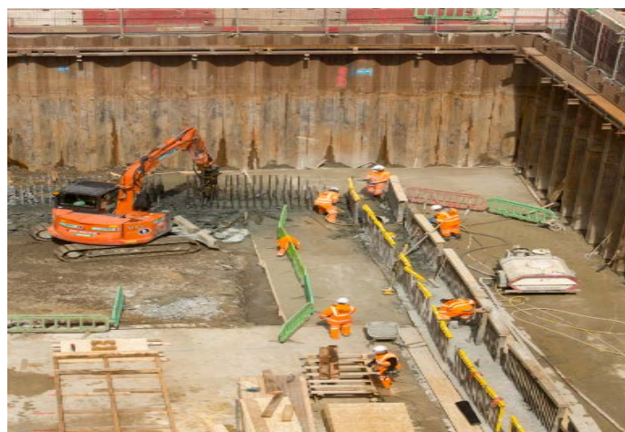
Image to show the excavator cropping the diaphragm wall
