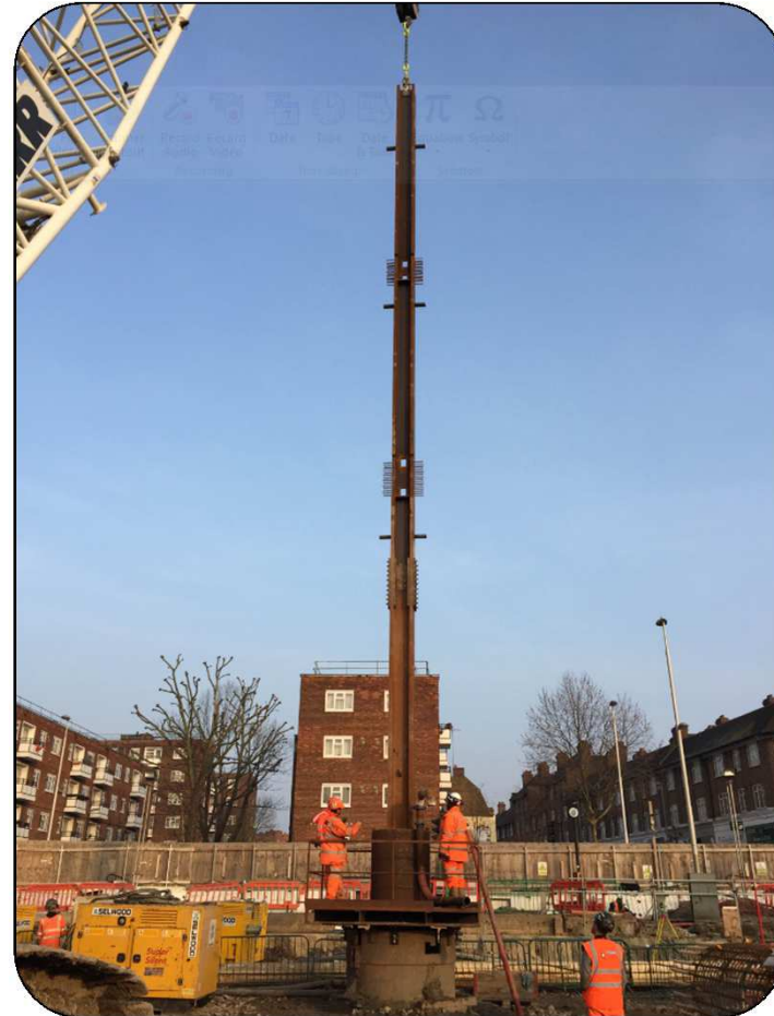
Plunge columns to be inserted in bearing piles
