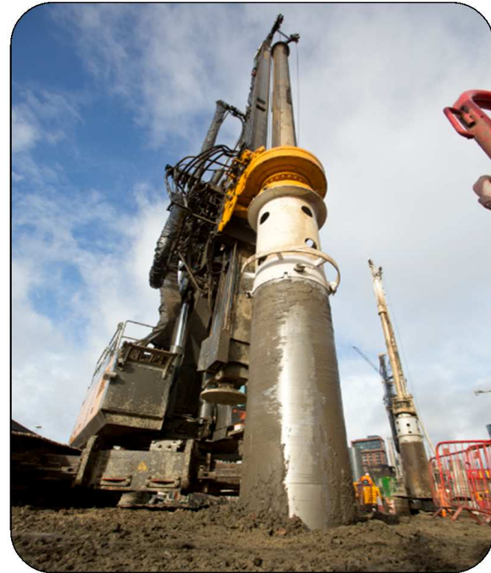
Removal of pile obstructions
