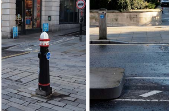
Bollard-mounted signs, to diagram 955 for a cycle route (left) and diagram 956 for shared use (right)
