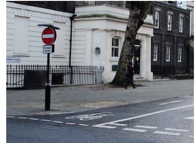
Area-wide authorisations issued in October 2011 made it possible to add an 'Except cycles' plate to a 'no entry' sign to permit contraflow cycling
