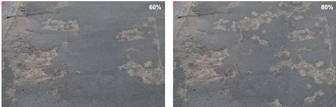
Figure 22: Bitumen fretting – bitumen users
