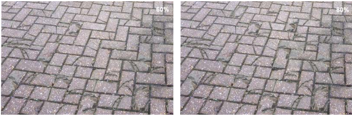
Figure 30: Blocks: Cracking – blocks users
