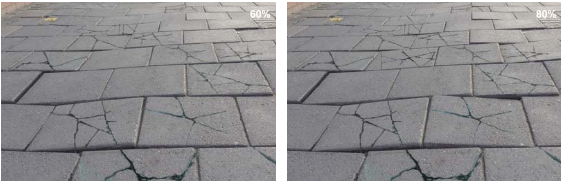
Figure 27: Flags: Cracked and depressed – all footway users
