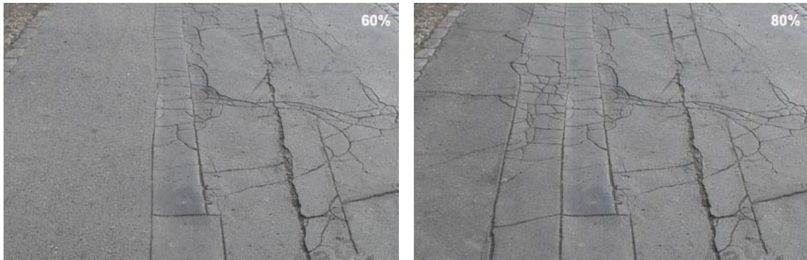
Figure 24: Bitumen: cracking– bitumen users
