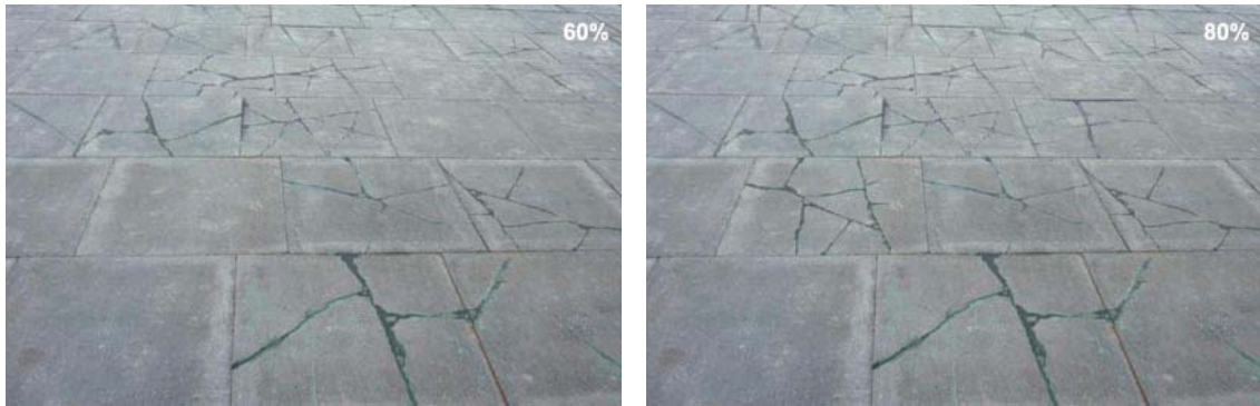
Figure 25: Flags: cracking – all footway users
