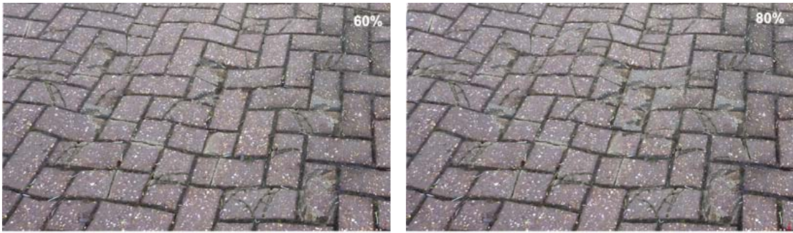
Figure 32: Blocks: Cracked and depressed – blocks users
