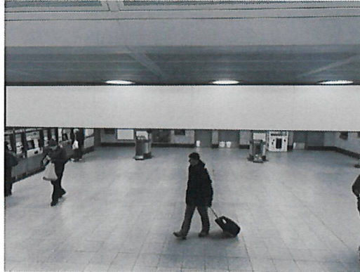
Overhead signage at entrance to ticket hall
