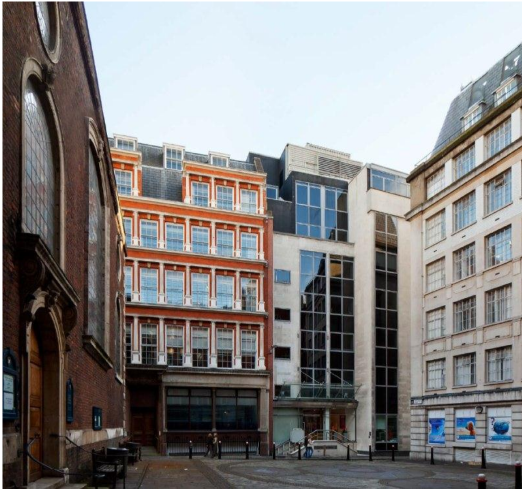
Figure 3.6: Existing View from Abchurch Yard Facing 20 Abchurch Lane
