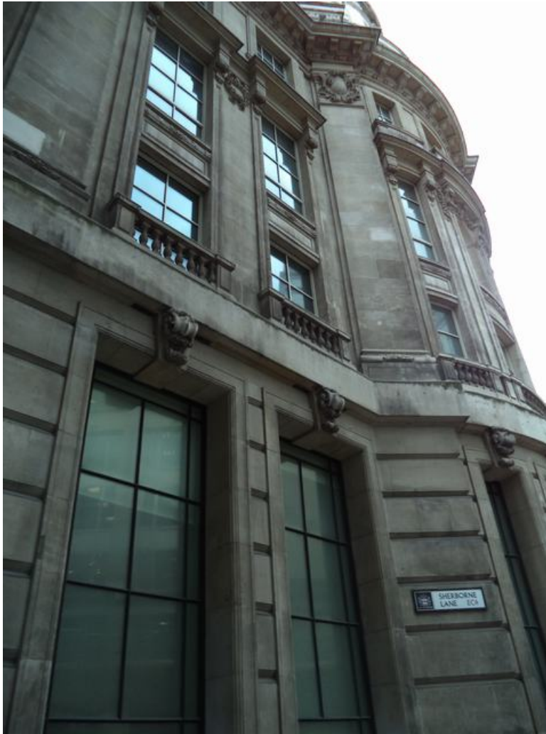
Photo 2: Section of Sherborne Lane elevation in the location of the largest predicted settlement
