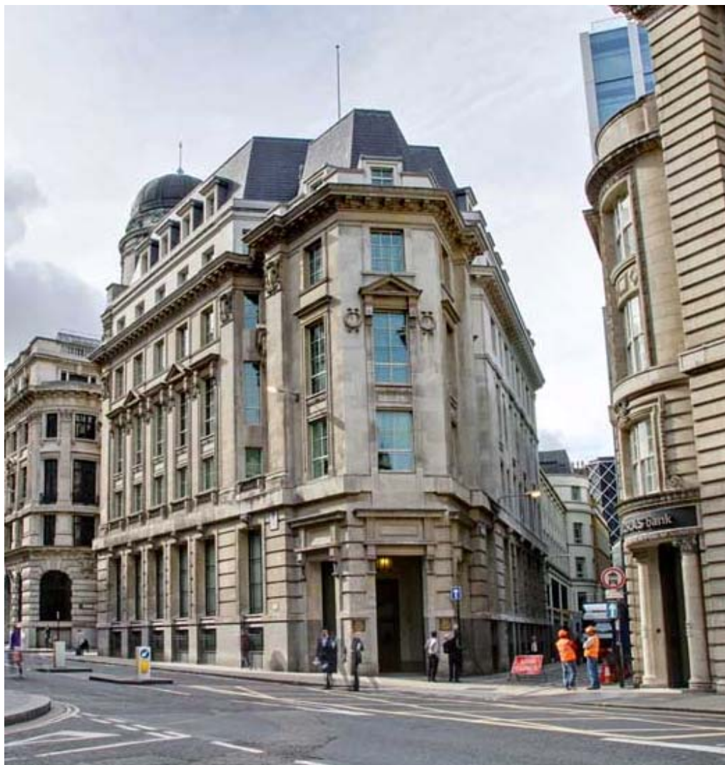
Photo 1: General view of 1 King William Street
