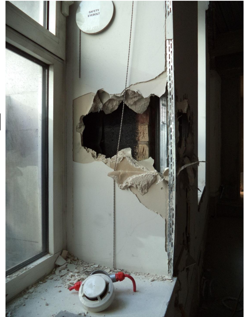
Current typical interior finish in area of proposed strengthening works, showing masonry external wall behind opened-up plaster during works undertaken by others
