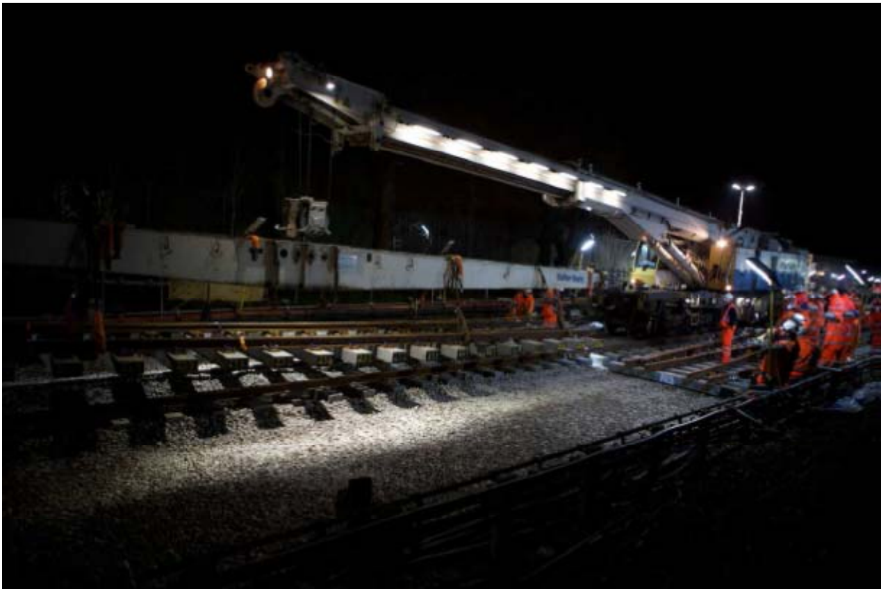
Modular points and crossings installation at Ruislip
