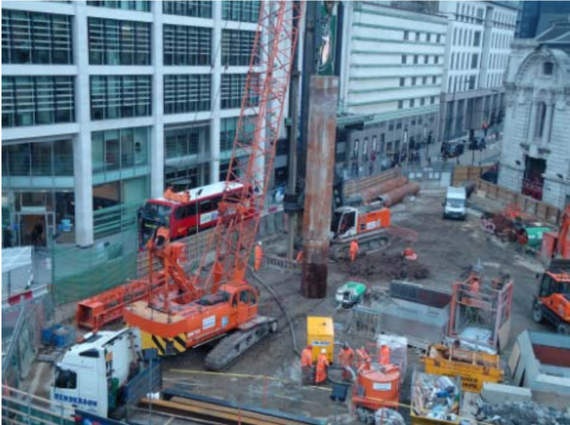
Victoria South Ticket Hall piling works
