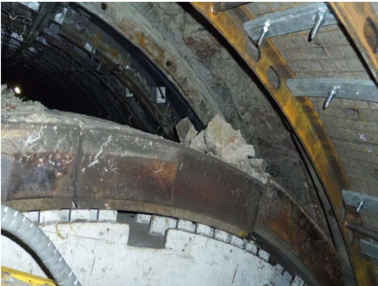
Shoulder tunnel segment being lowered
