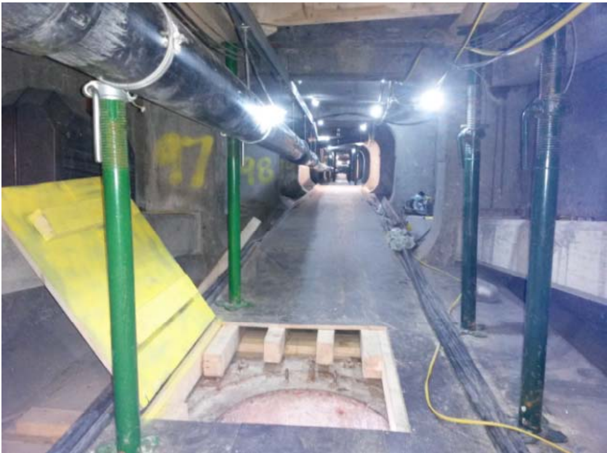
Inside Hammersmith Flyover
