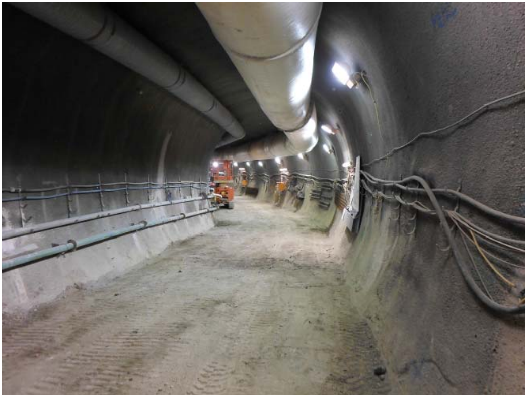
Victoria station tunnelling
