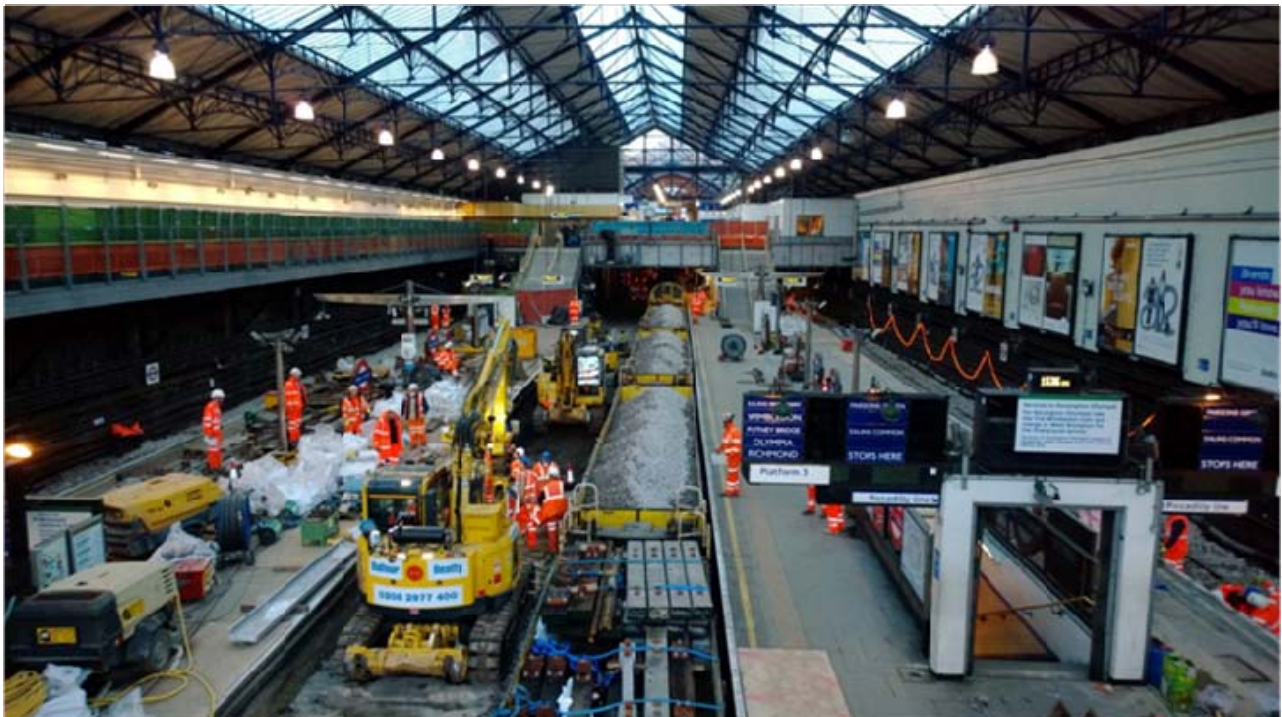
Ballasted Track Renewal at Earl's Court
