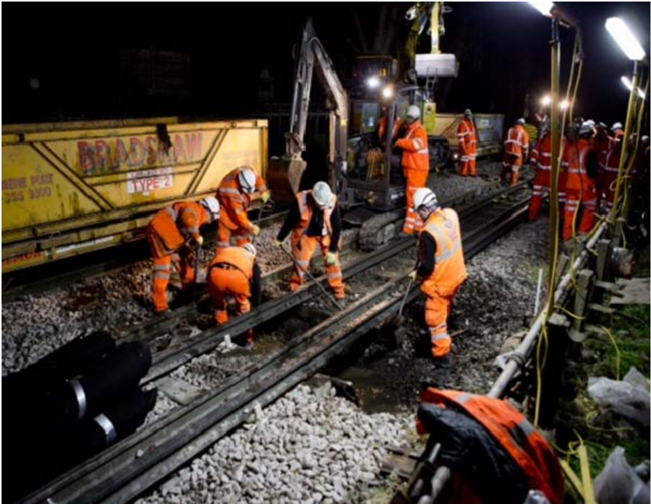
Overnight midweek track re-ballast works on the Central line
