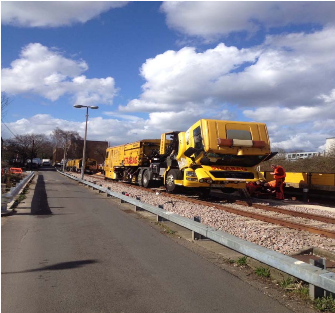
New Strabag milling machine:TDU rail grinding project
