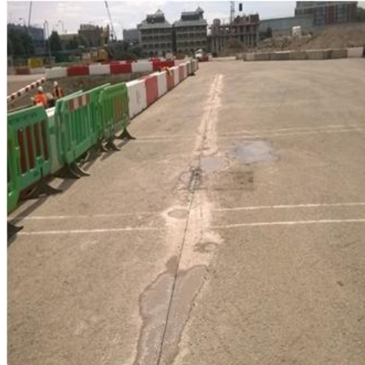
Removal of obstructions left behind from previous industrial use
