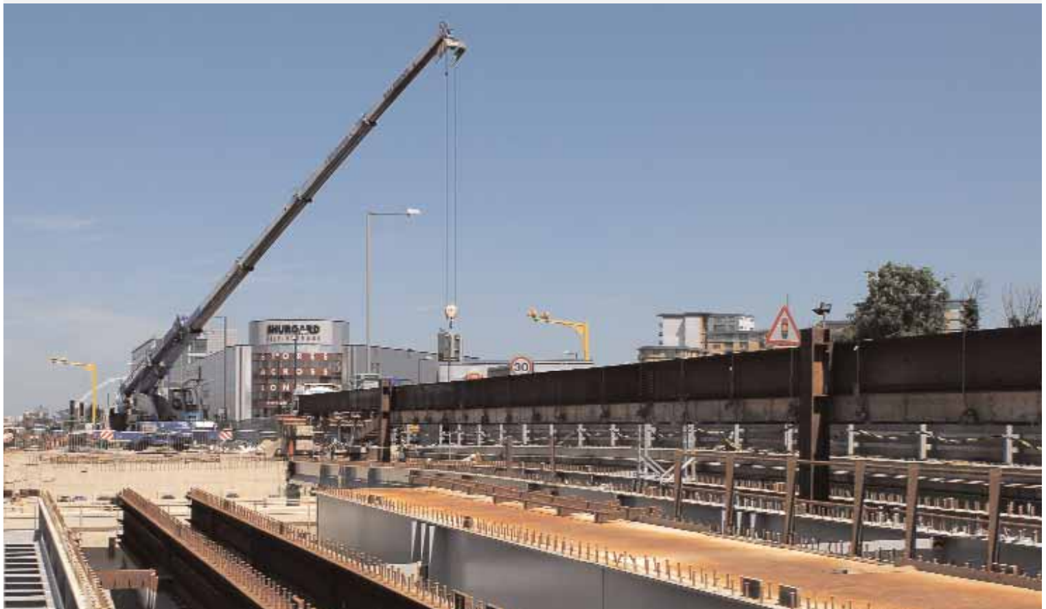
The A40 Western Avenue Bridge replacement scheme, which will create two new roads over rail bridges and secure the route over the railway for the next 120 years. It will also deliver significant improvements to cycling and walking facilities in the area
