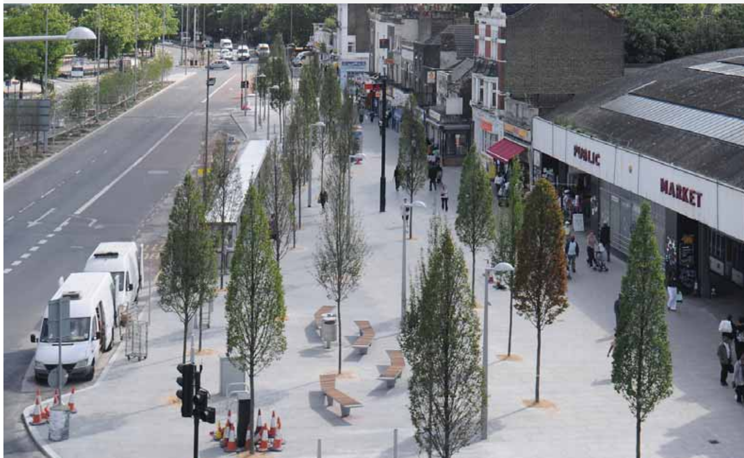
Improvements already delivered as part of the Woolwich town centre project
